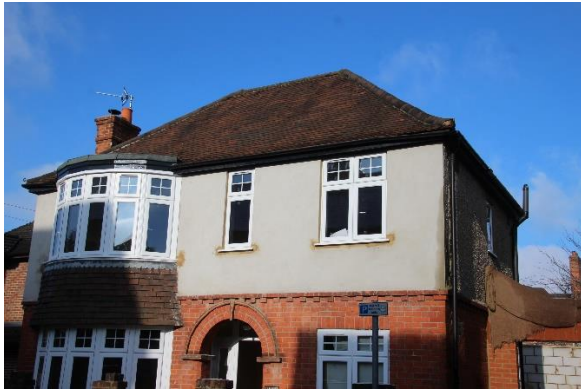
1. 18 Goldsmid Road from the south-east
