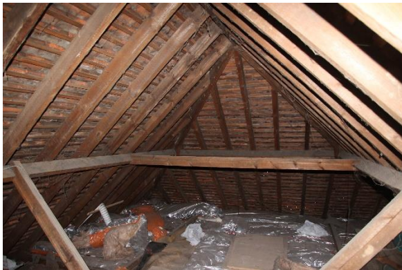
5. Main roof space looking north-east
