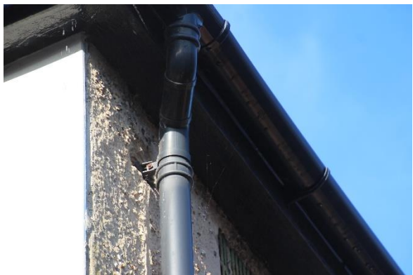
4. Well-sealed soffits and render
