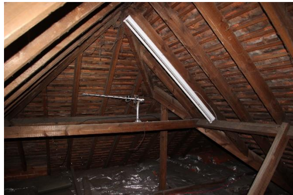
6. Main roof space looking north-west
