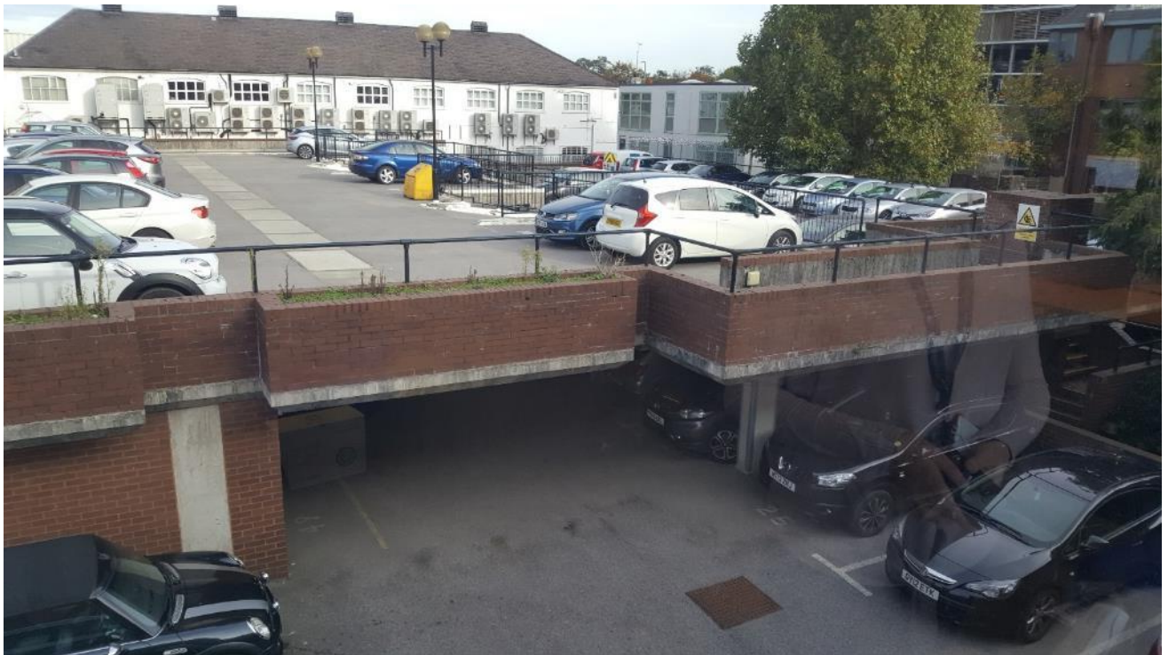
Photograph 4: Multi-storey car parking in the north-west of the site
