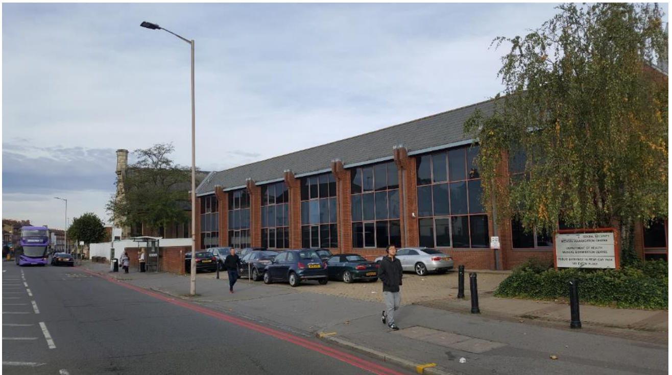
Photograph 8: Oxford Road elevation with mature tree on-site (to the right of the picture)
