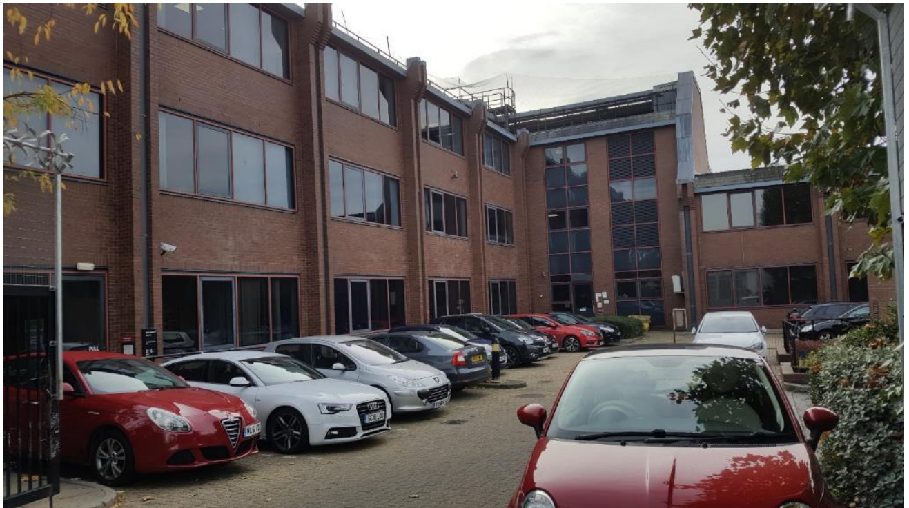
Photograph 1: The office building on-site from north to south-east
