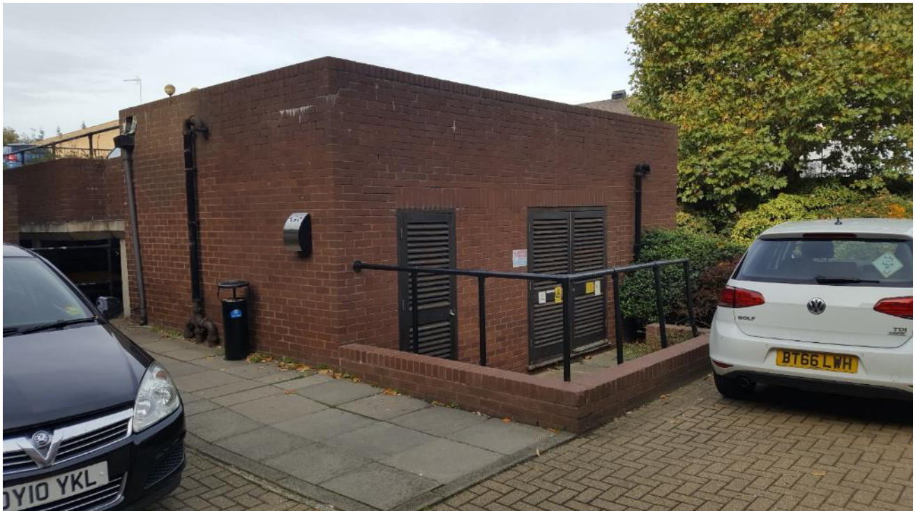
Photograph 12: Electrical plant building in the centre of the site, adjacent to the car park
