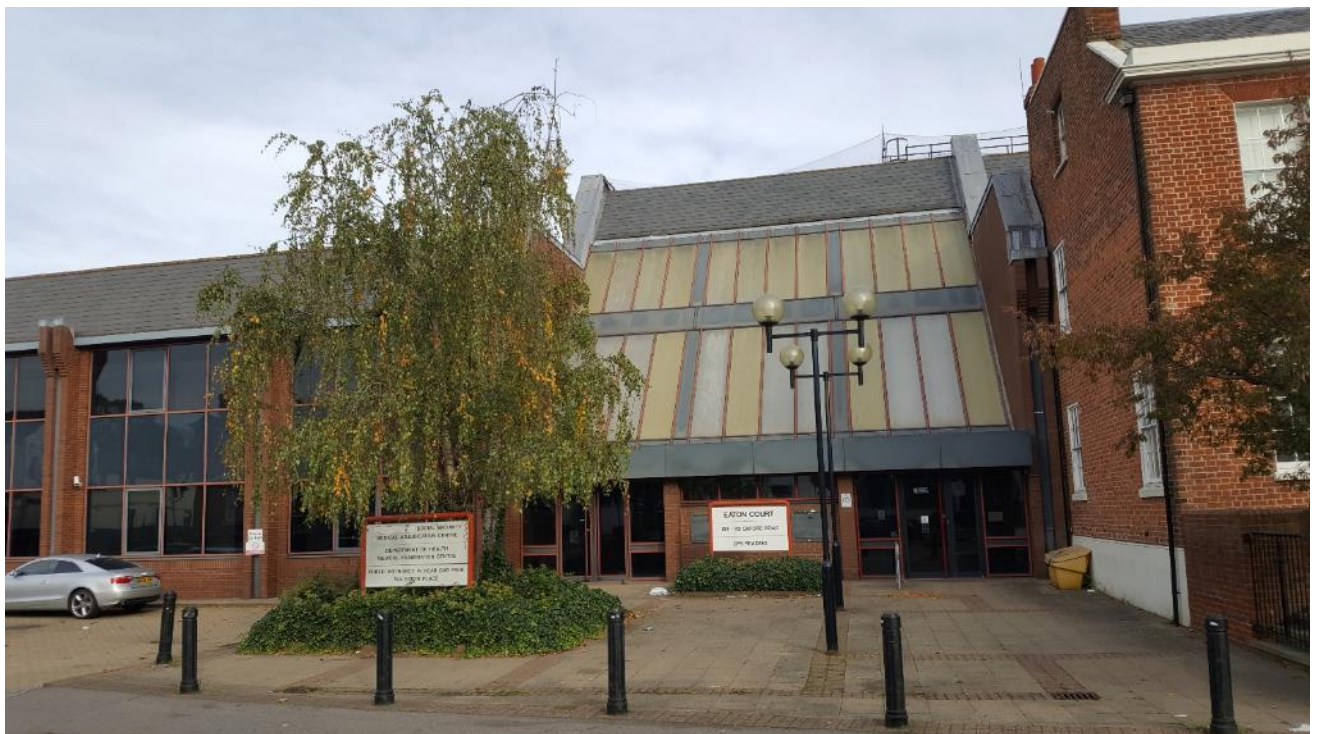
Photograph 2: View of the office building entrance from the south
