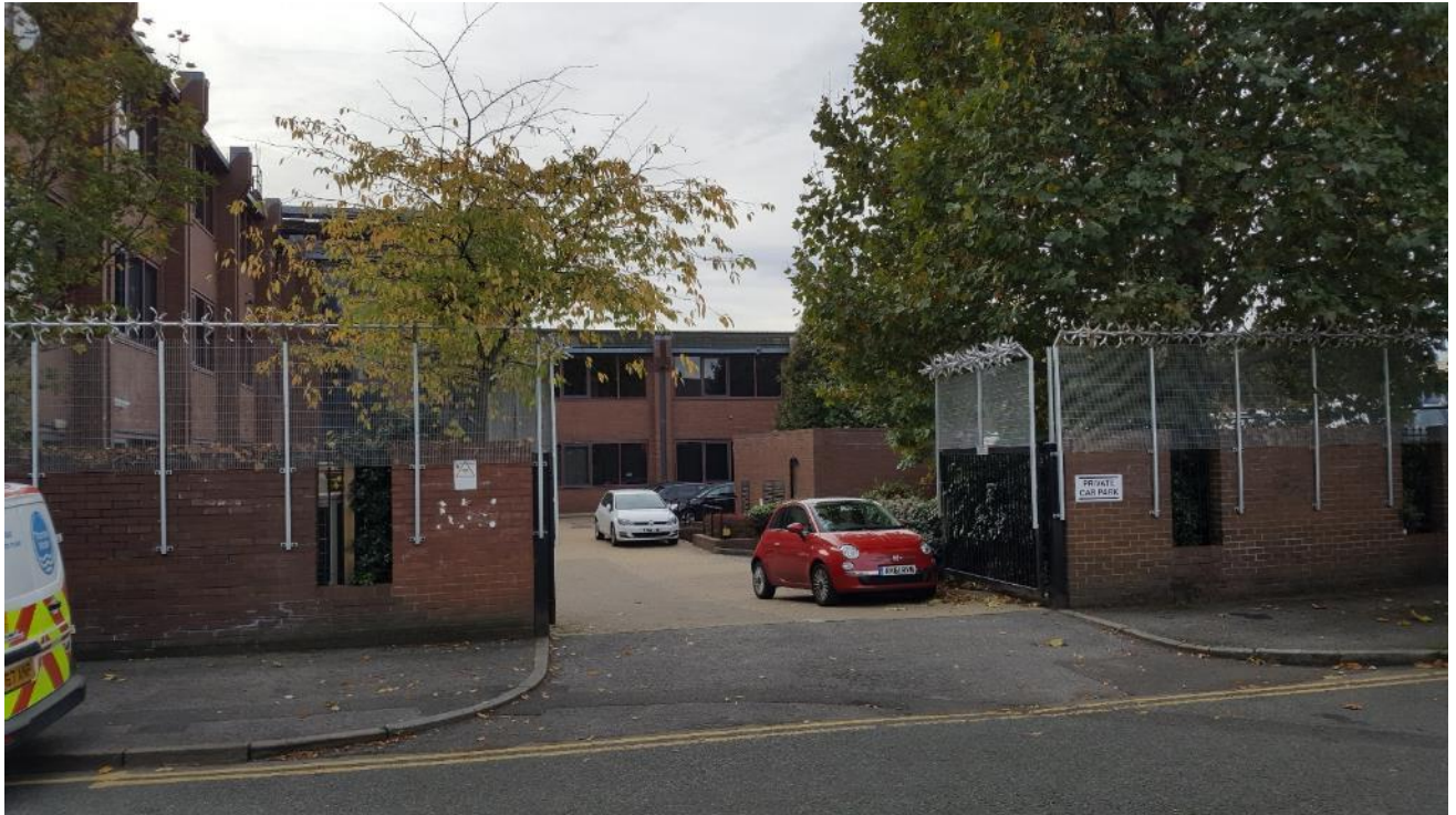
Photograph 3: Service road leading onto the north-west of the site. Mature tree evident in right foreground.
