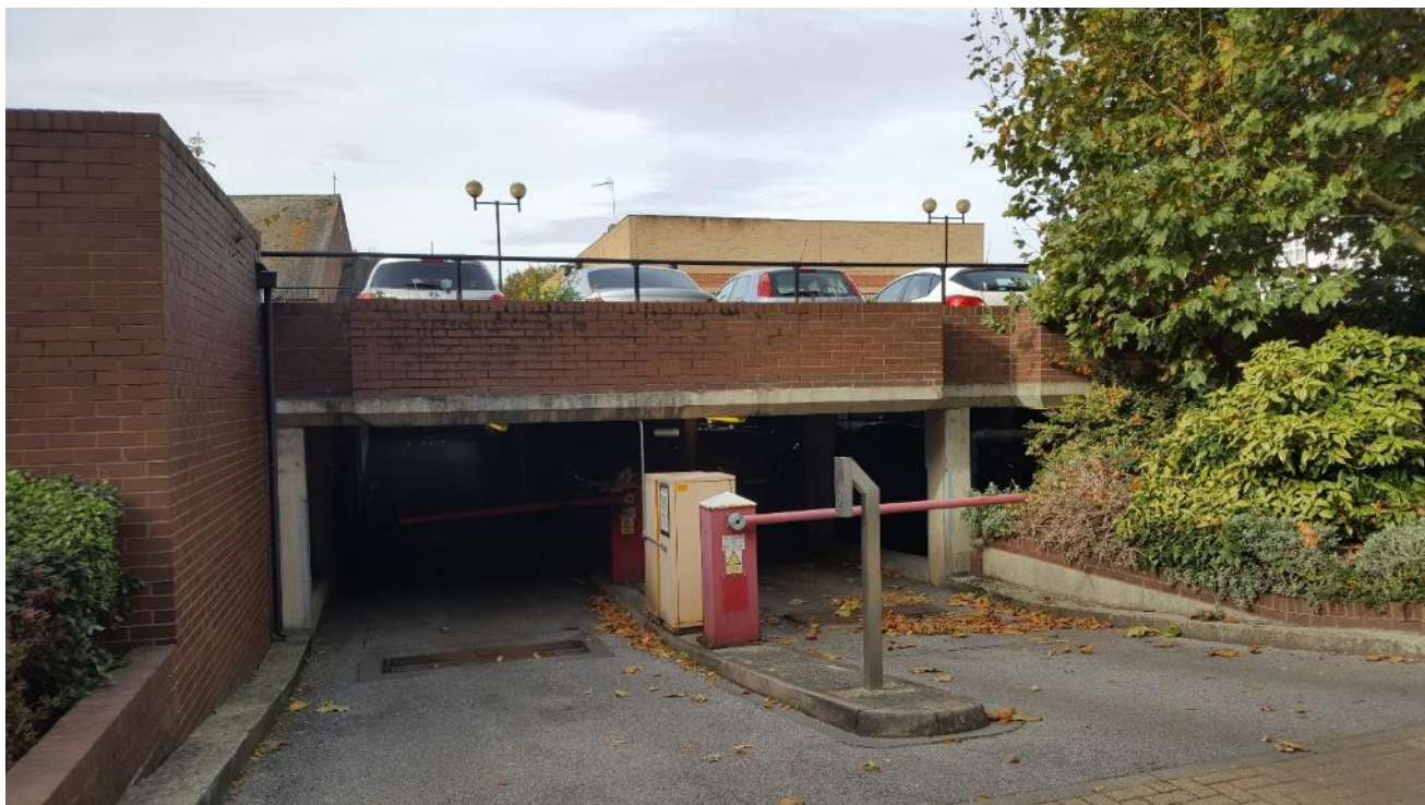
Photograph 5: Entrance and exit to undercroft level of the car park in the north-west of the site
