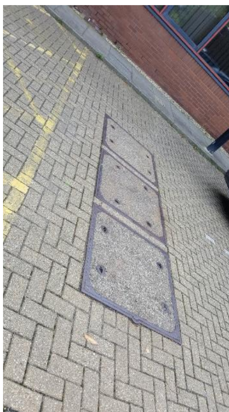
Photograph 14: Access covers overlying an oil/water separator (interceptor) in the centre of the site
