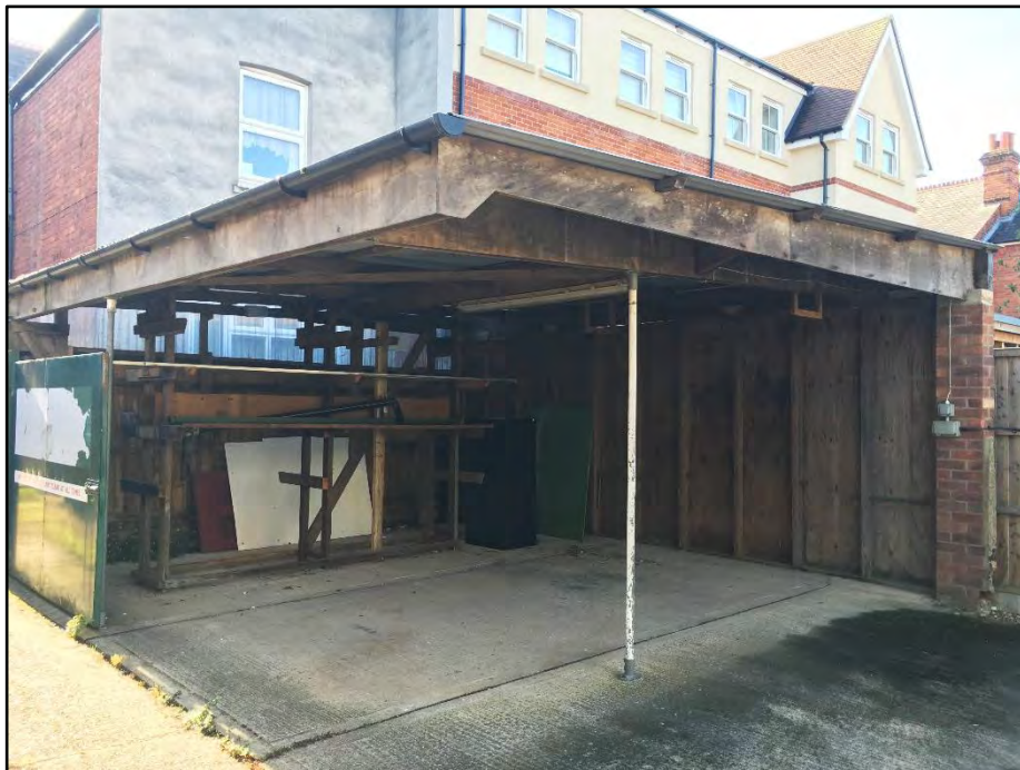
Figure 4: Photograph of Open Sided Building Onsite
