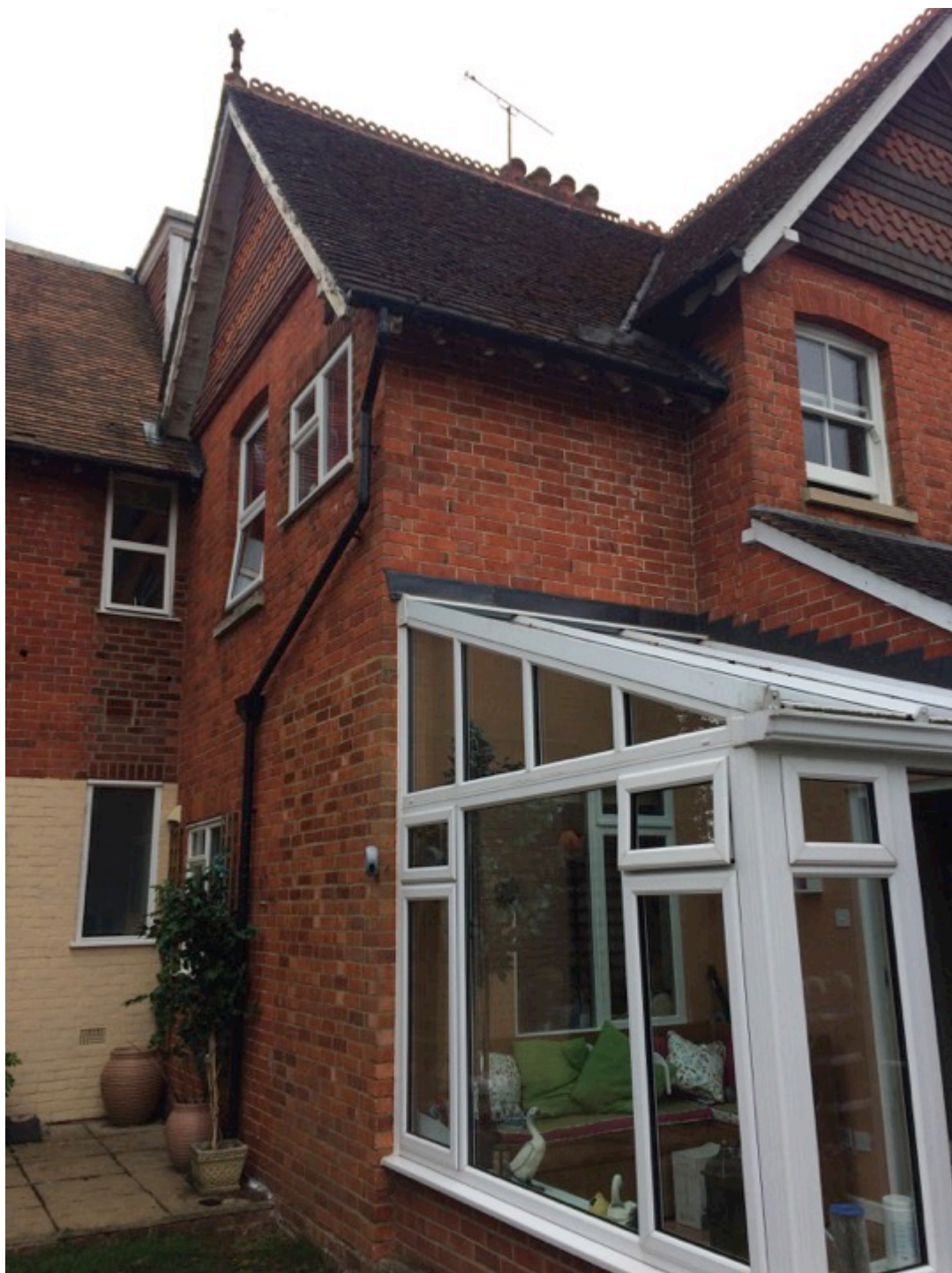
Figure 2: Existing rear UPVC conservatory to be demolished
