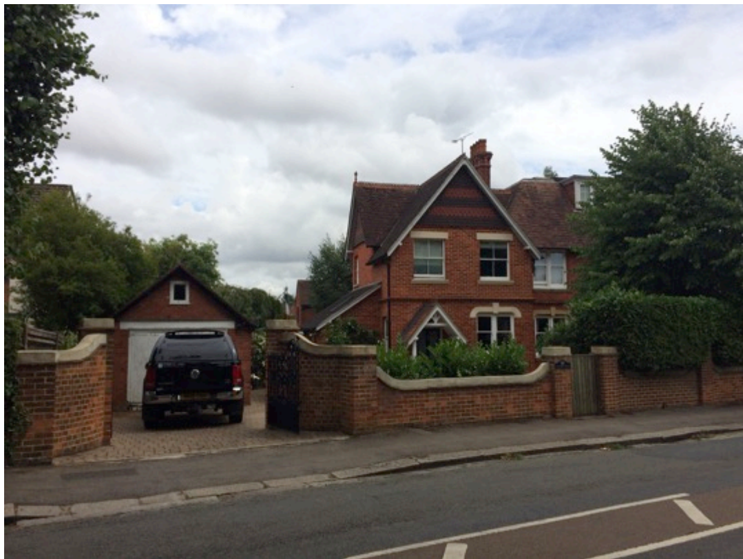
Figure 1: Front (West) Elevation of 48 Albert Road, showing the existing tile hanging gable, garage to the north and scalloped wall detail to the front
