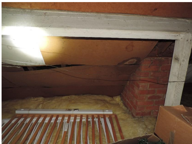
Plate 6. General view internal void space.
