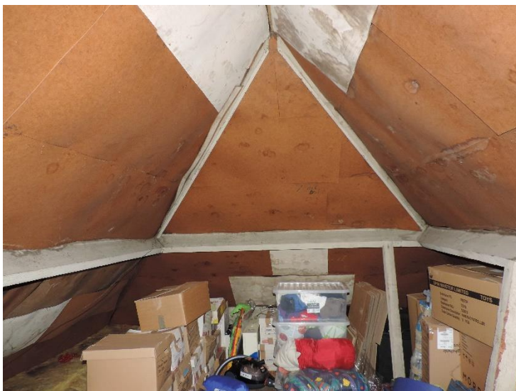
Plate 5. General view of internal void space.
