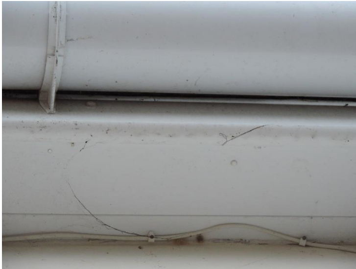
Plate 4. Typical view of the soffit and fascia boards.
