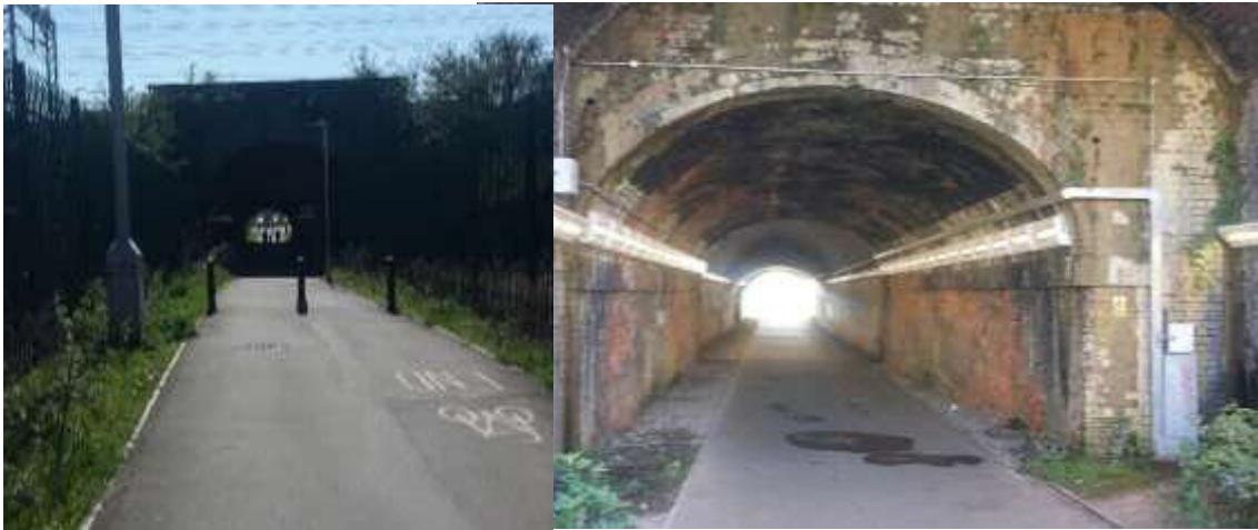
Photo 3.3 – Railway underpass between Napier Road and Kenavon Drive
