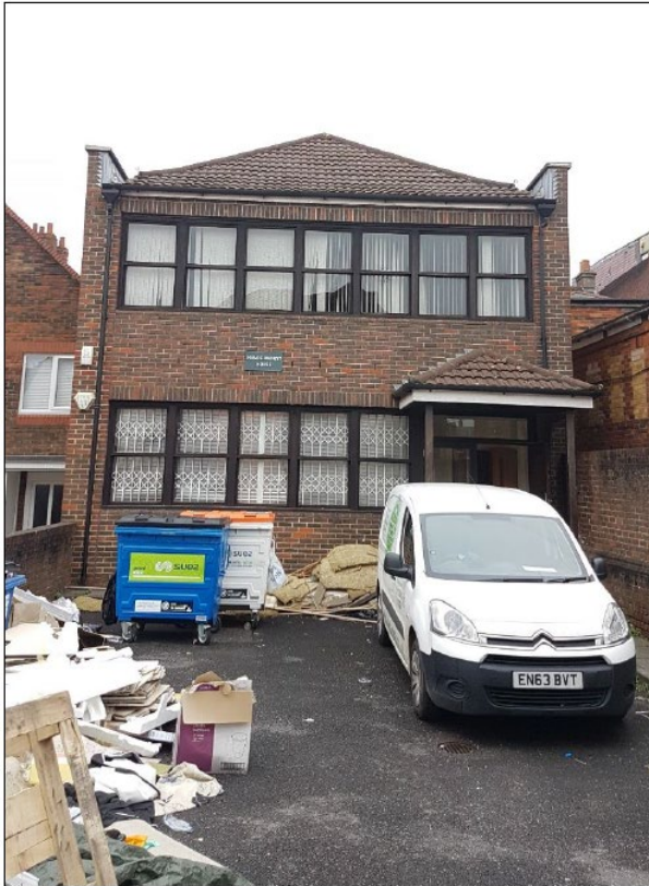
Plate 1. Building 1b (view: east)
