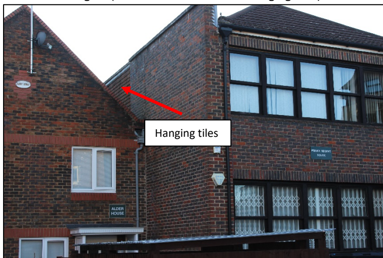
Plate 2. Building 1b (northern elevation with hanging tiles)
