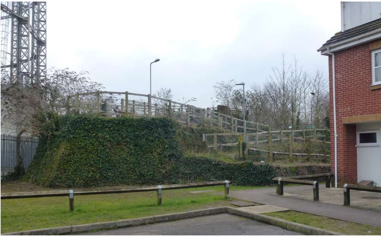
View access to the bridge link from Kennet Walk
