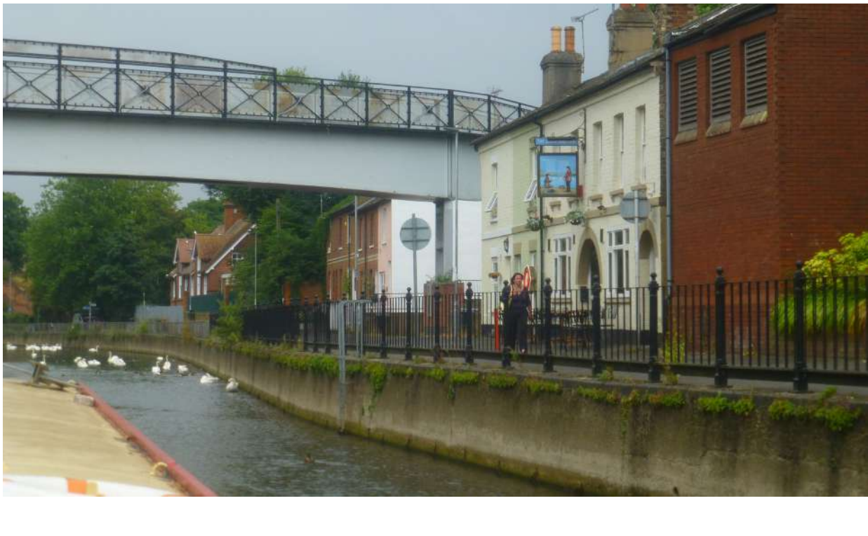
View of the existing bridge from the River Kennet
