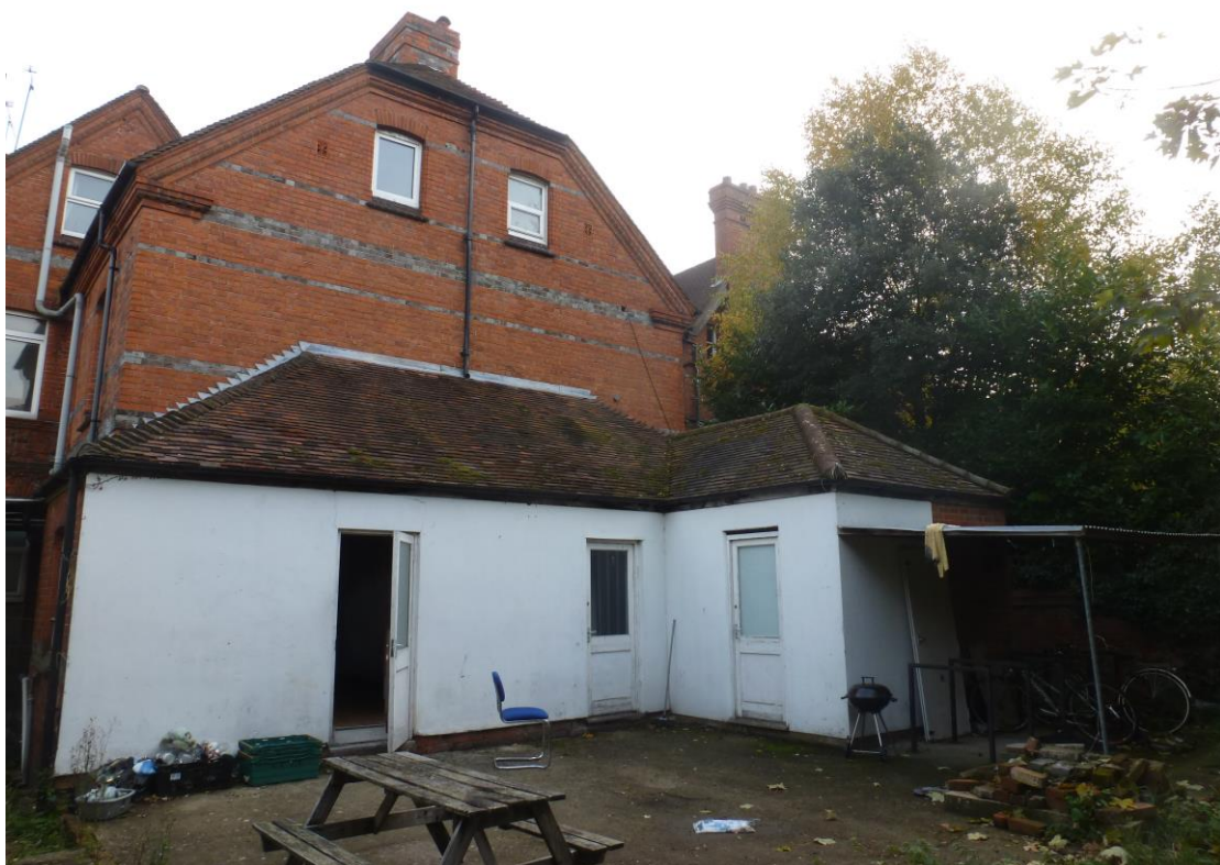
Fig.8: Rear view photograph illustrating existing poor quality extension to be demolished
