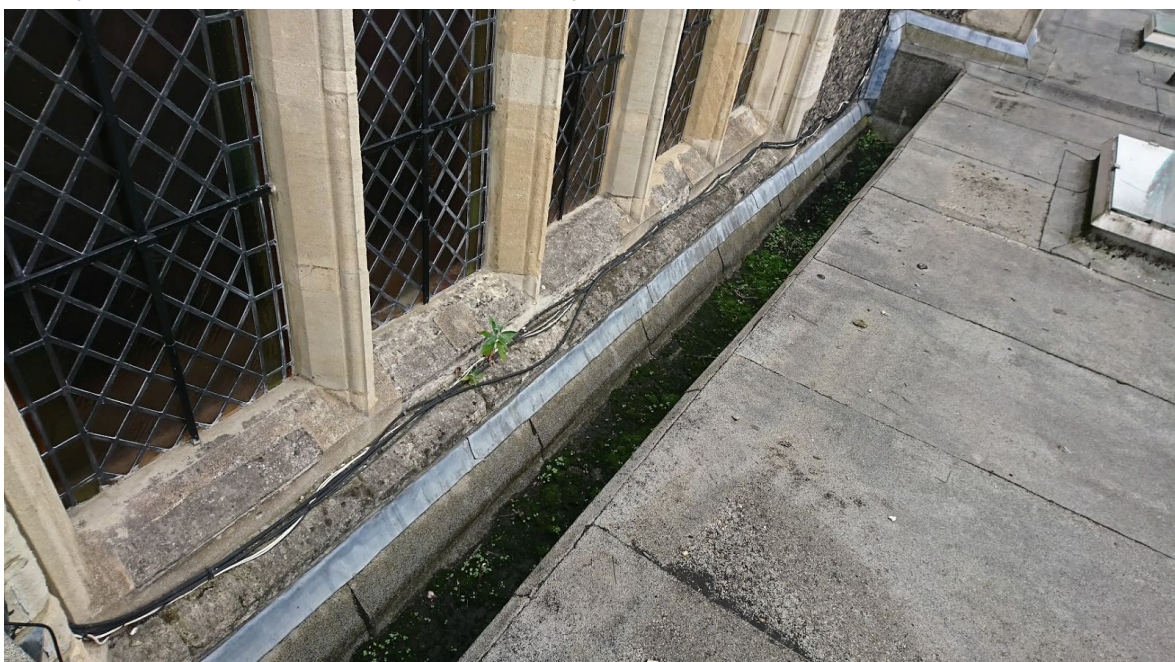
Below: junction of 1972 roof with renewed 14th century west window
