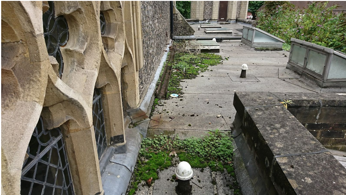
Above: flat roof to 1972 north link and west end extension
