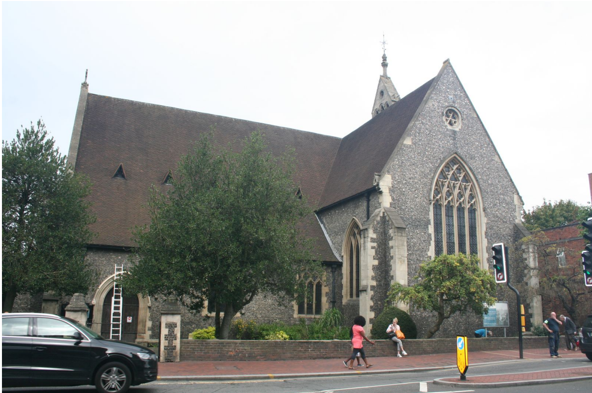
Above: south elevation of the friary church, looking north
