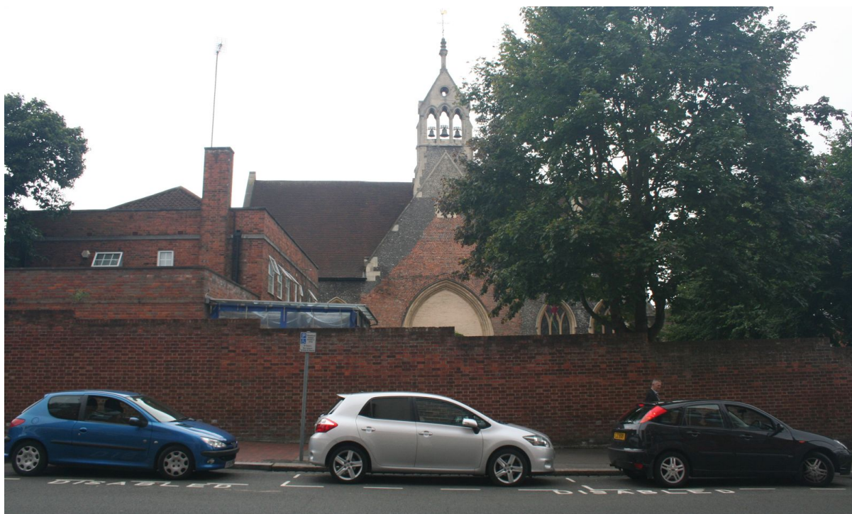
Above: east elevation from Greyfriars Road; 64 Friar Street, the old rectory and current church owned nursery, is on the left. The bell turret is Woodman's.
