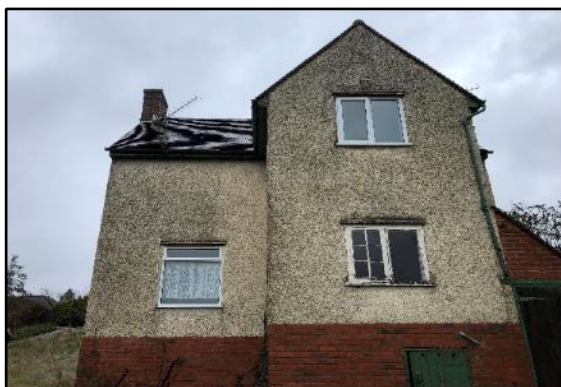
Photo 40: building 203 coal shed
