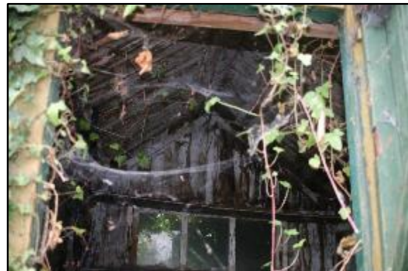
Photo 35: building 201a interior
