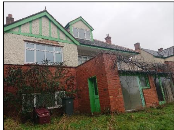
Photo 33: building 201 south elevation
