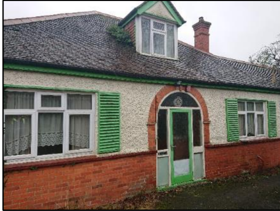
Photo 30: building 201 – northern elevation
