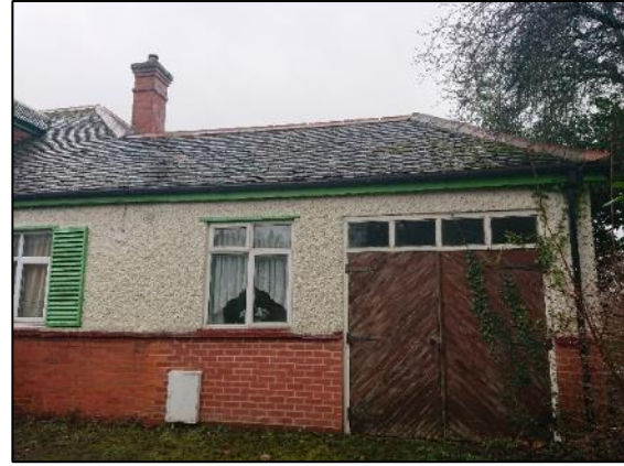
Photo 31: building 201 – northern elevation
