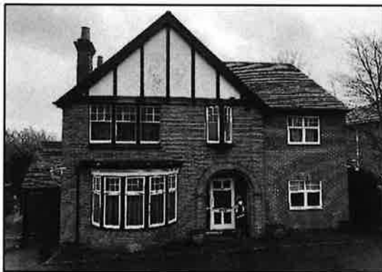
Photo 21: Building 199 front (north)
