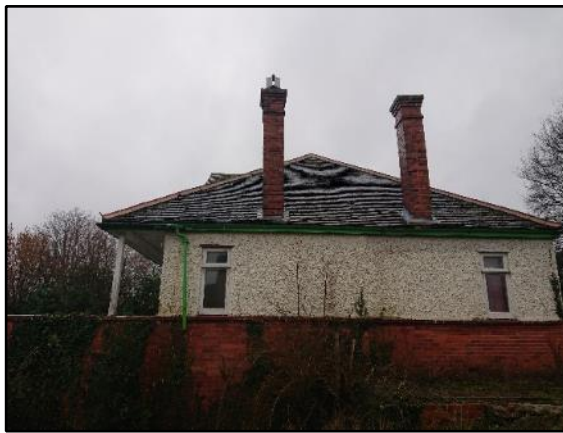
Photo 32: building 201 eastern elevation
