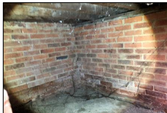
Photo 41: building 203 coal shed
