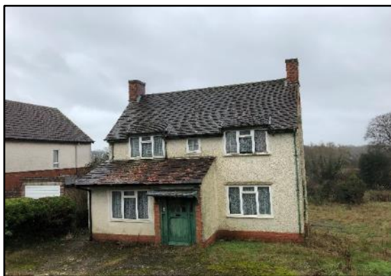
Photo 38: building 203 north elevation
