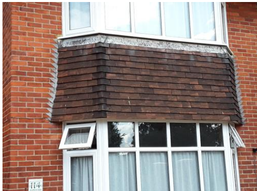
hanging tiled wall within front elevation
