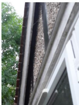
open soffits on the rear elevation providing potential access and crevice spaces
