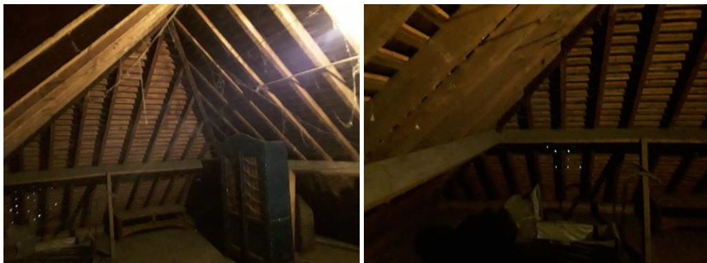
internal loft space – visible light noted within the exposed tiles
