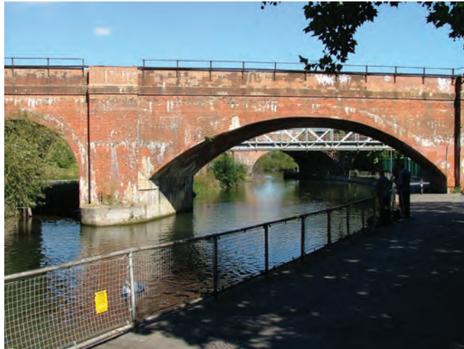
1. View of listed railway bridge
