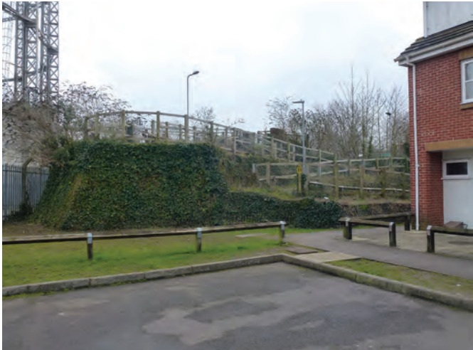
10. View of ramp connection to pedestrian bridge
