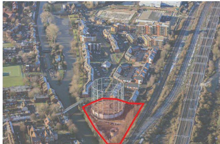
Aerial view from east
