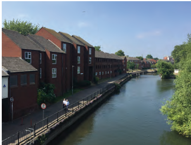
1. View from pedestrian bridge, looking south
