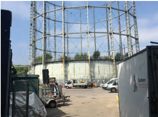
4. View of existing gas holder from within the site
