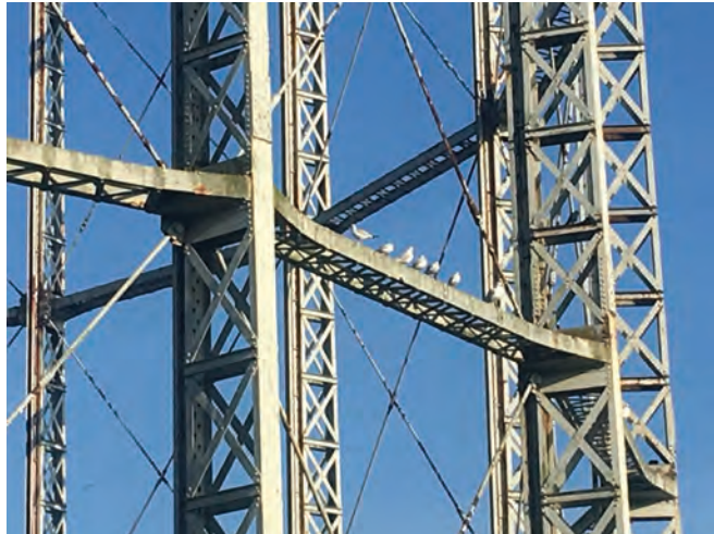
Detail of existing structure
