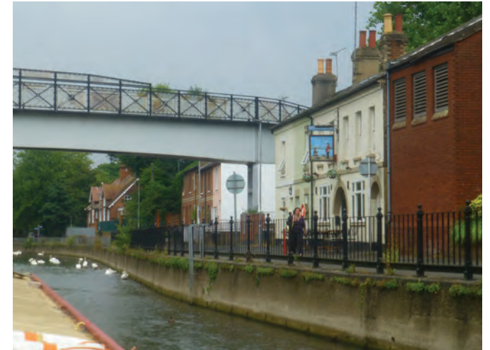
2. View of pedestrian bridge
