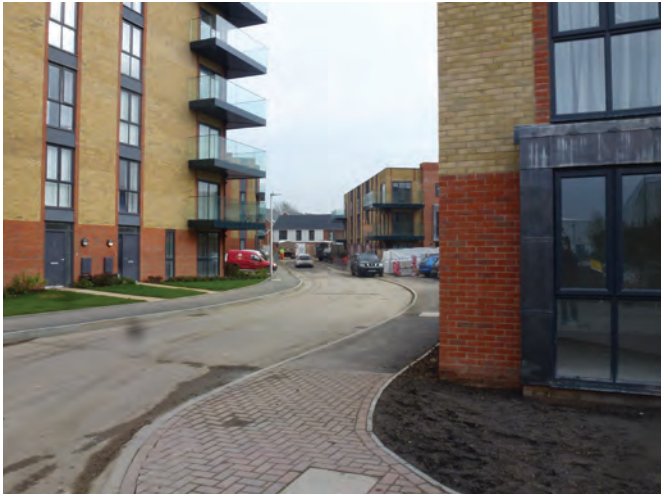
3. View from Robert Parker Road, looking east
