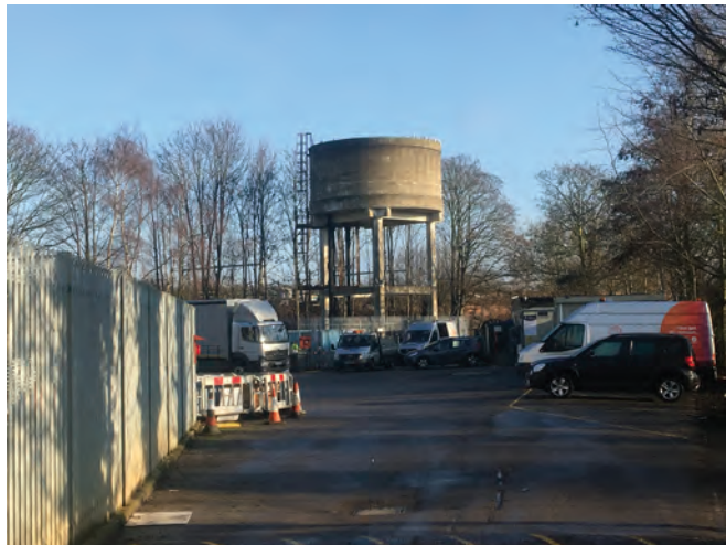
5. View of existing water tower
