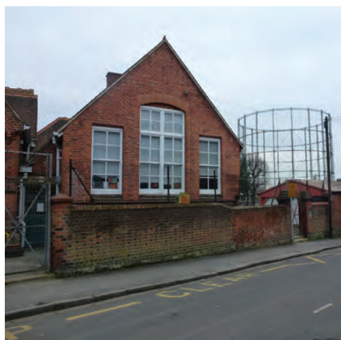
New Town Primary School (Grade II listed)
