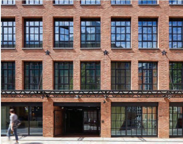
Curtain Hotel, Dexter Moren Associates
