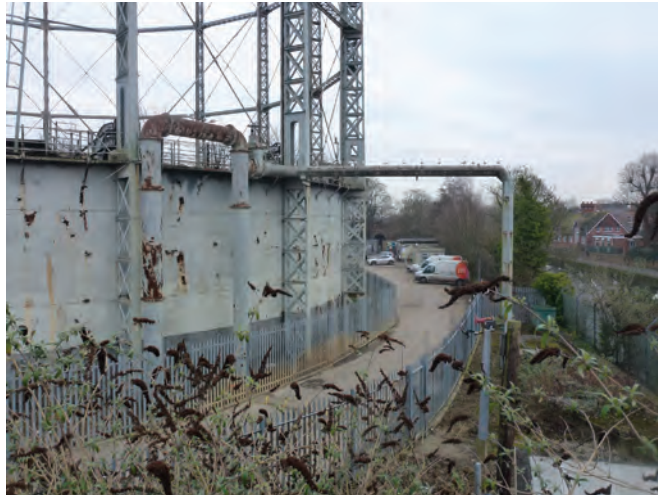
2. View from pedestrian bridge over access road, looking east
