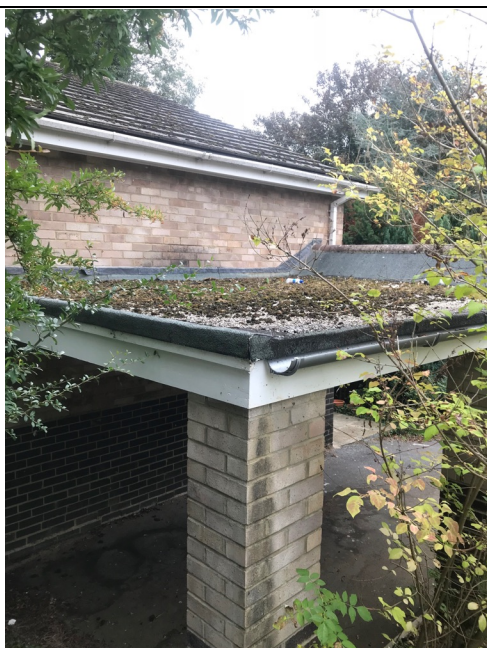
Photo 9 – Western carport No.46
