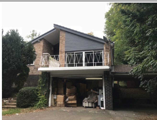
Photo 8 – South-western elevation of No. 46
