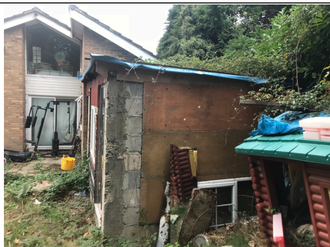
Photo 2 – Garage to rear of No.48 to be demolished
