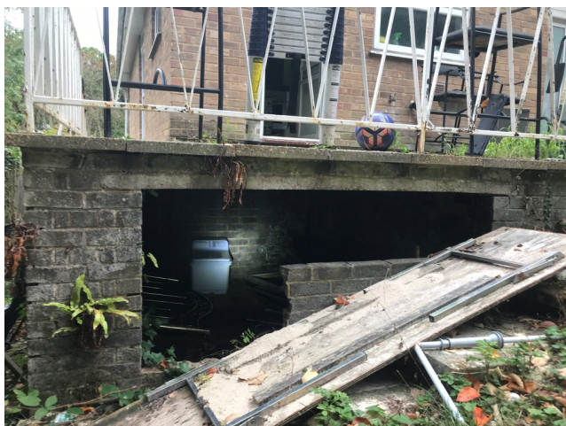
Photo 3 – Area under the rear patio of No.48
