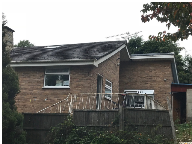
Photo 4 – View of roof of No.48
