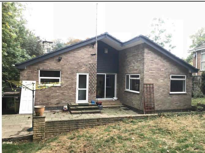
Photo 7 – North-eastern elevation of No. 46
