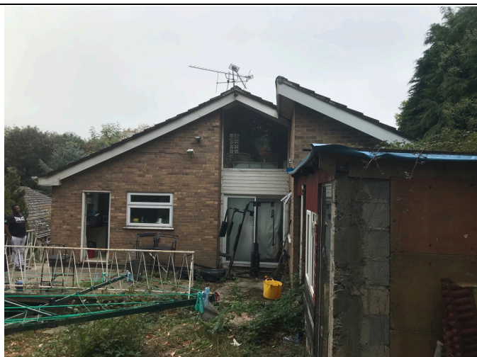
Photo 1 – North-eastern elevation of No. 48
