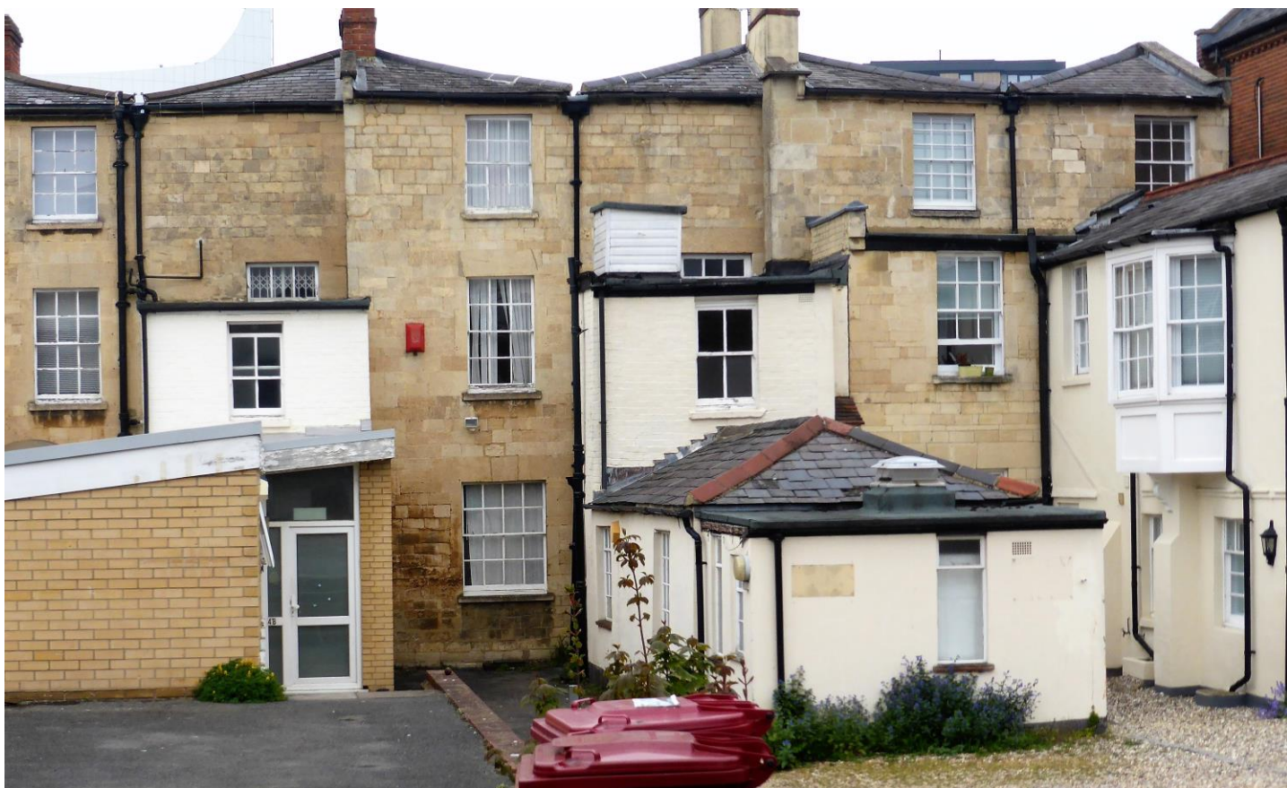
PHOTO 1. Unsightly rear office toilet block and staff room with flat roofed kitchen extension above and a water tank above that. The proposal replaces this jumbled excrescence with a self-contained single-storey pitched-roofed extension whose design and materials are much more sympathetic and in accord with the character of the original listed terrace.
