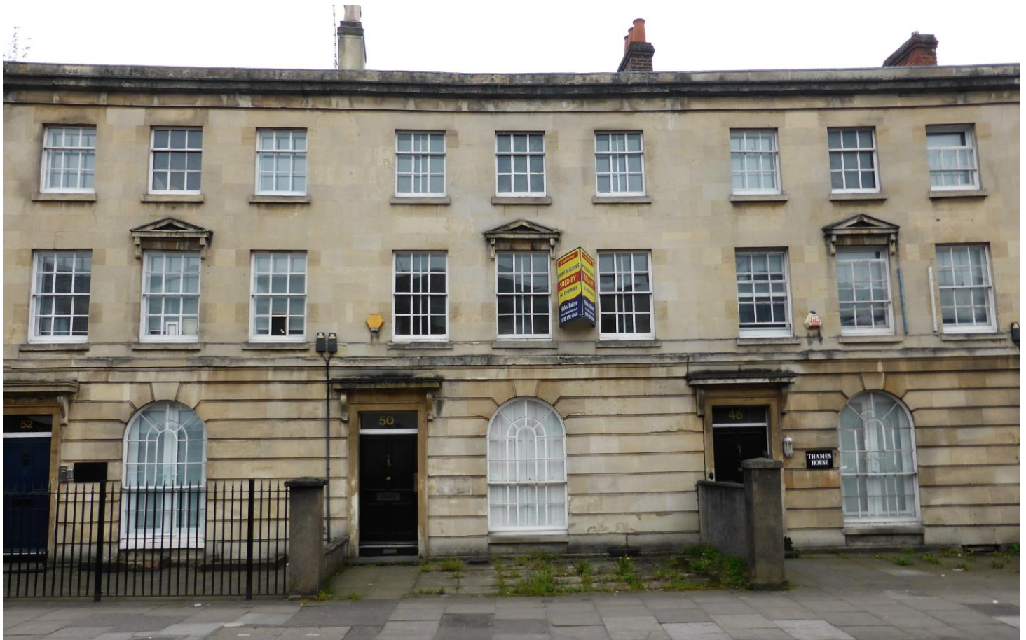
PHOTO 1. The frontage of 50 Queens Road lies dead centre. It is a 3 storey building constructed of Bath stone ashlar. It and all the crescent to the right are GII GV Listed Buildings.
