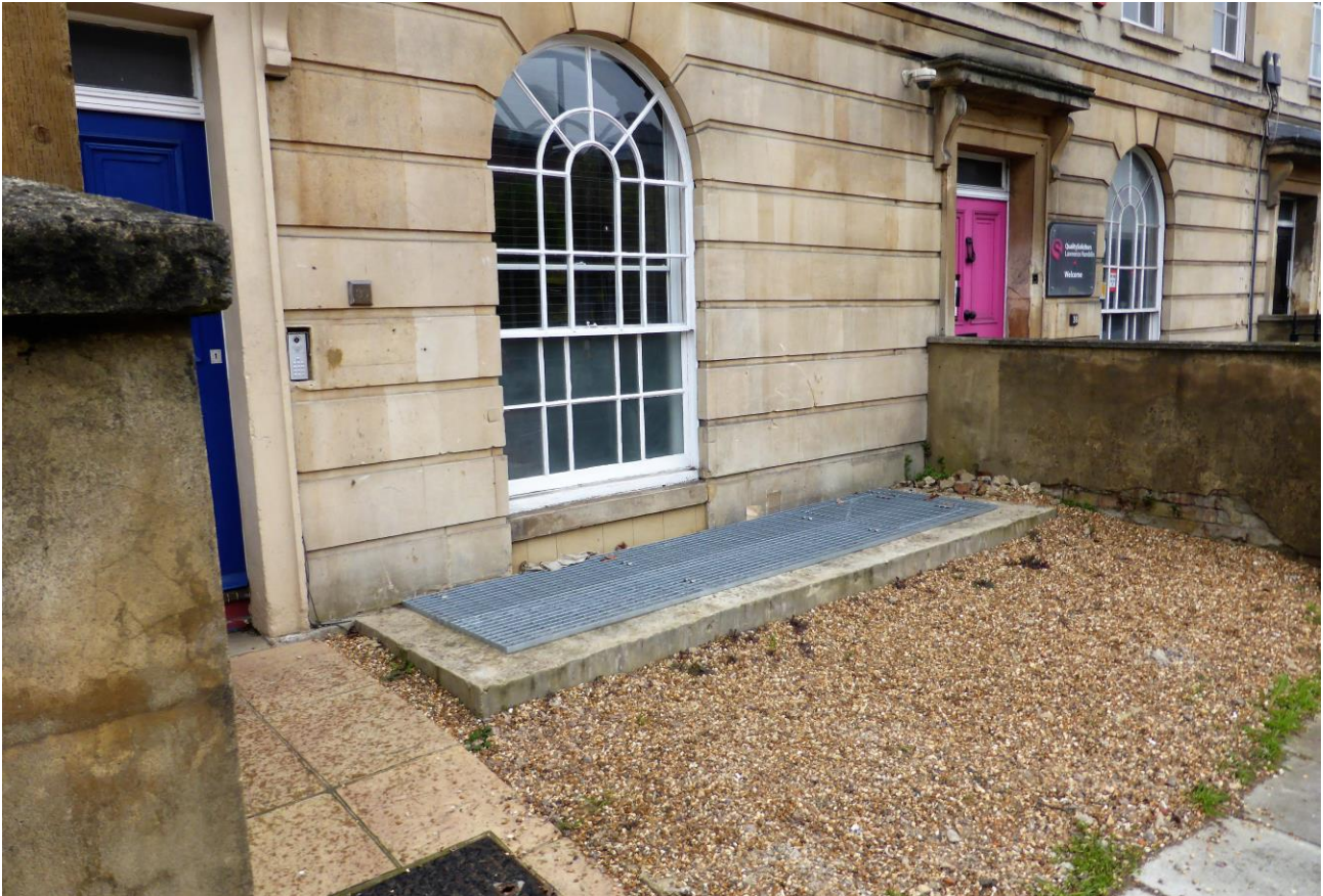
PHOTO 4. Example of approved frontage lightwell similar to that proposed.
