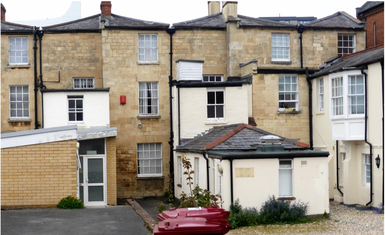
PHOTO 2. Contextual photograph taken April 2019 looking north showing the GII (GV) listed 50 Queens Road in the centre. Number 48 lies to the left (west) number 50 lies to the right (east). The unsightly rear office toilet block and staff room to be demolished is evident. The proposal replaces this jumbled excrescence with a self-contained single-storey pitched-roofed extension whose design and materials are much more sympathetic and in accord with the character of the original listed terrace.
