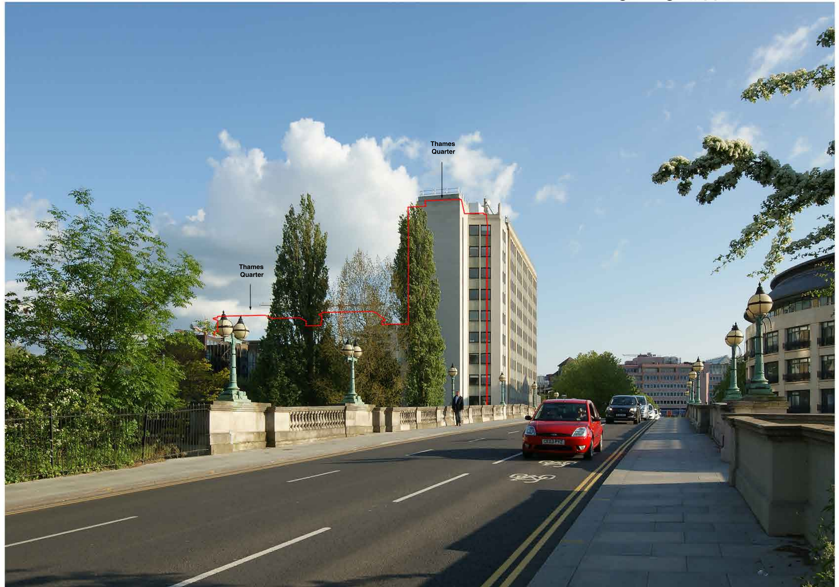
From the north-west of the bridge.
