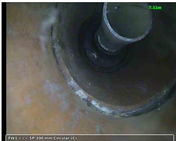
20190529-160652-snap0002.jpg, 00:00:40, 7.11 m Finish node type, manhole, reference number: SP
