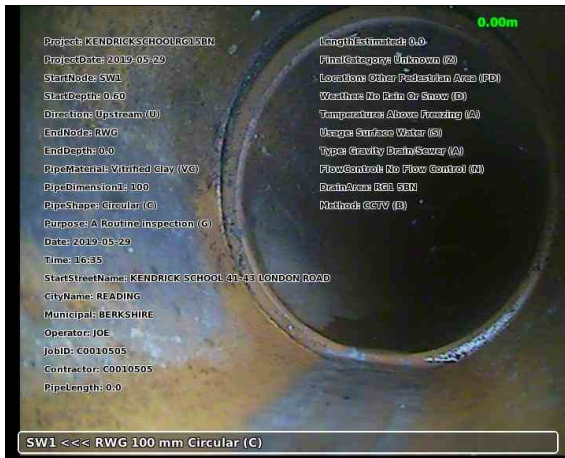
20190529-163553-snap0000.jpg, 00:00:00, 0.00 m Start node type, manhole, reference number: SW1
