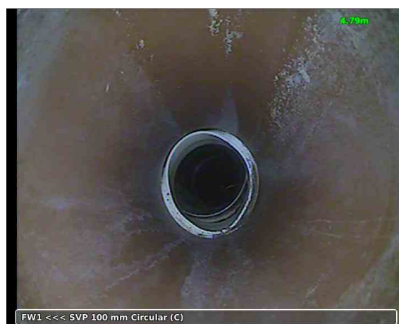
20190529-160922-snap0003.jpg, 00:00:37, 4.79 m Finish node type, manhole, reference number: SVP
