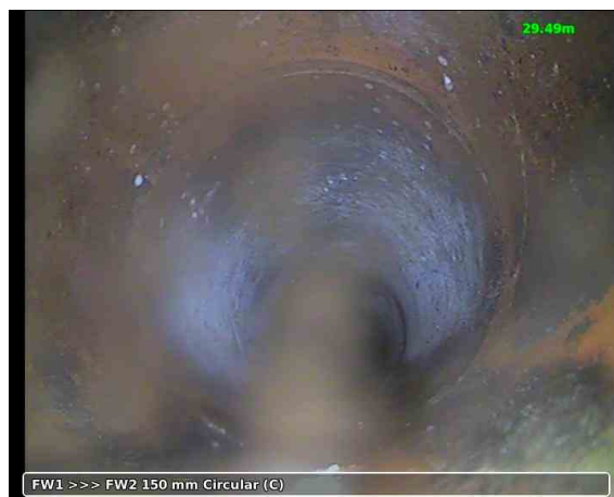
20190529-161316-snap0001.jpg, 00:01:19, 29.49 m Line deviates down
