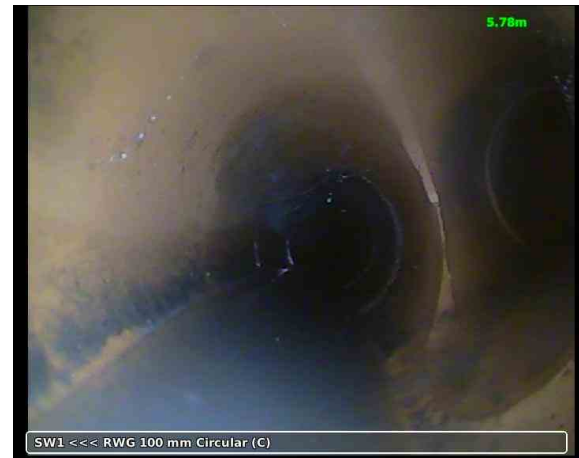
20190529-163553-snap0002.jpg, 00:00:35, 5.78 m Junction, at 03 o'clock, diameter: 100 mm, RWP
