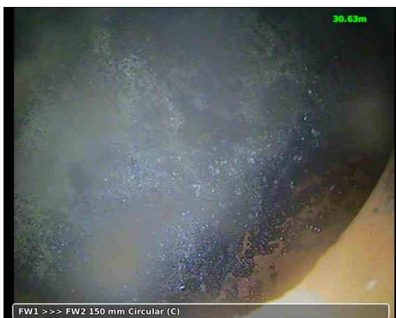
20190529-161316-snap0002.jpg, 00:01:30, 30.63 m Finish node type, manhole, reference number: FW2
