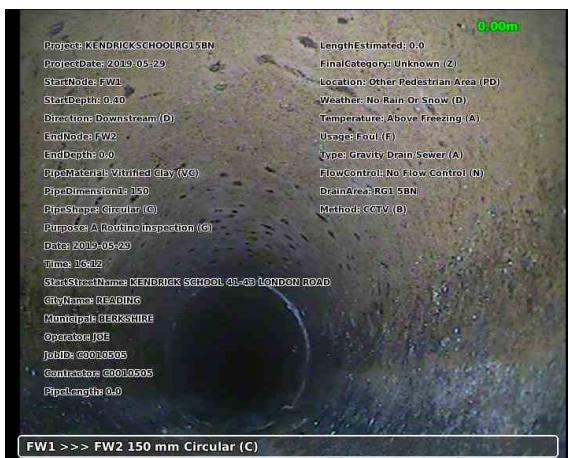
20190529-161316-snap0000.jpg, 00:00:01, 0.00 m Start node type, manhole, reference number: FW1
