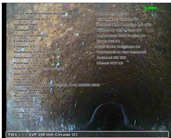
20190529-160922-snap0000.jpg, 00:00:01, 0.00 m Start node type, manhole, reference number: FW1
