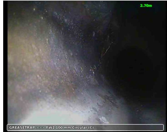
20190529-155647-snap0001.jpg, 00:00:28, 2.70 m Finish node type, manhole, reference number: FW1
