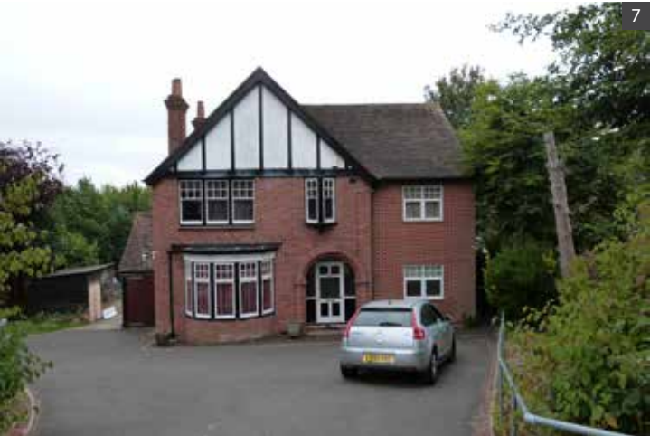
View of 201 Henley Road
