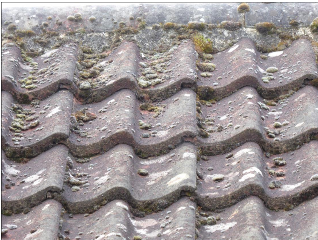
Figure 11. Close fitting composite roof tiles. 66 Chapel Hill, Tilehurst. 26.03.19
