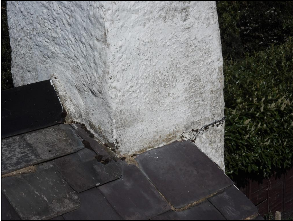
Figure 5. Close fitting tiles to chimney breasts, 66 Chapel Hill, Tilehurst. 26.03.19
