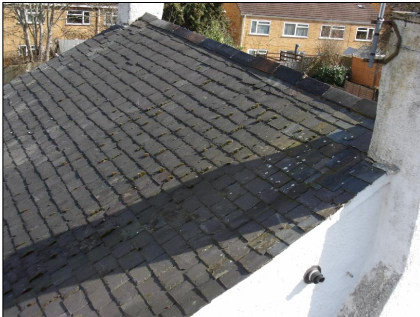
Figure 4. Main roof covering, 66 Chapel Hill, Tilehurst. 26.03.19
