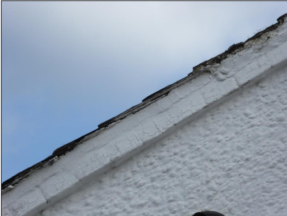
Figure 6. Example of sealed verges/fascia, 66 Chapel Hill, Tilehurst. 26.03.19
