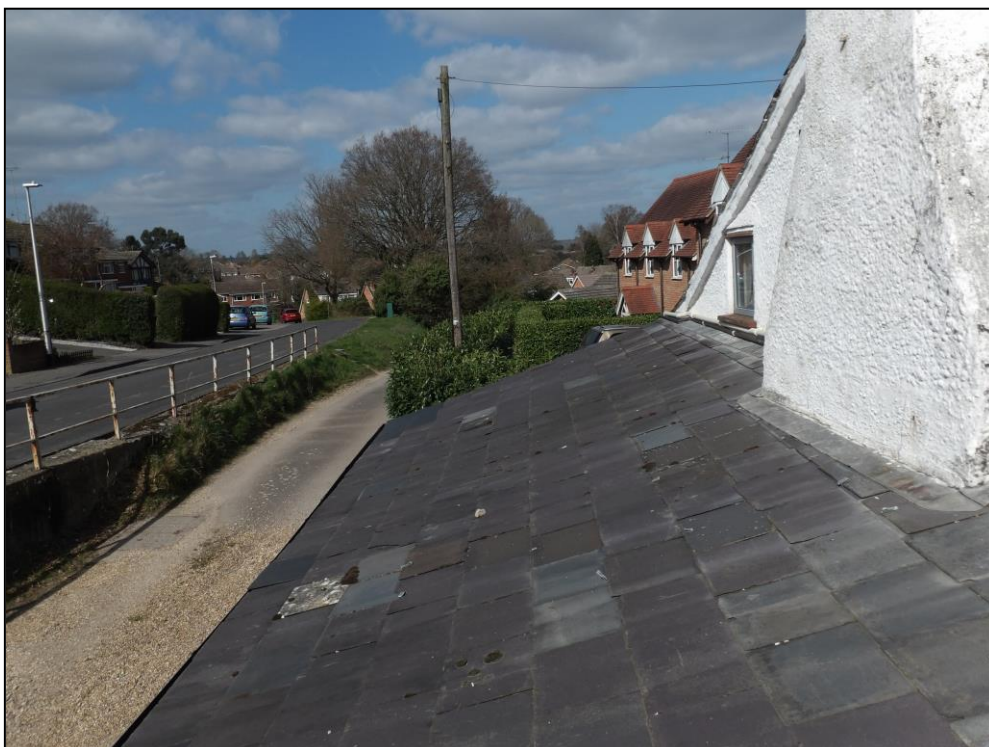
Figure 8. West side element with close fitting slate tiles and lead flashing. 66 Chapel Hill, Tilehurst. 26.03.19
