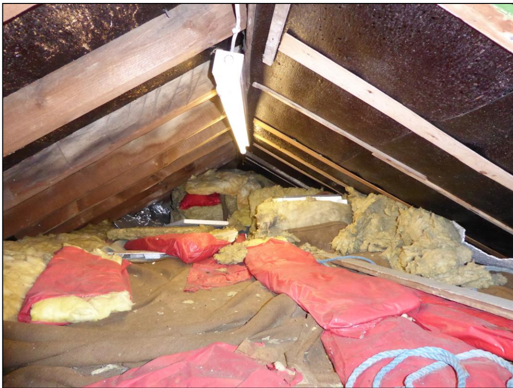
Figure 14. Example of loft space, 66 Chapel Hill, Tilehurst. 26.03.19
