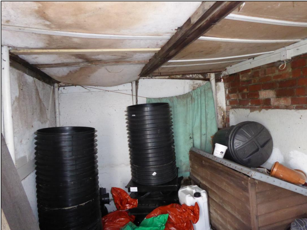
Figure 16. Internal view of outbuilding at 66 Chapel Hill, Tilehurst. 26.03.19
