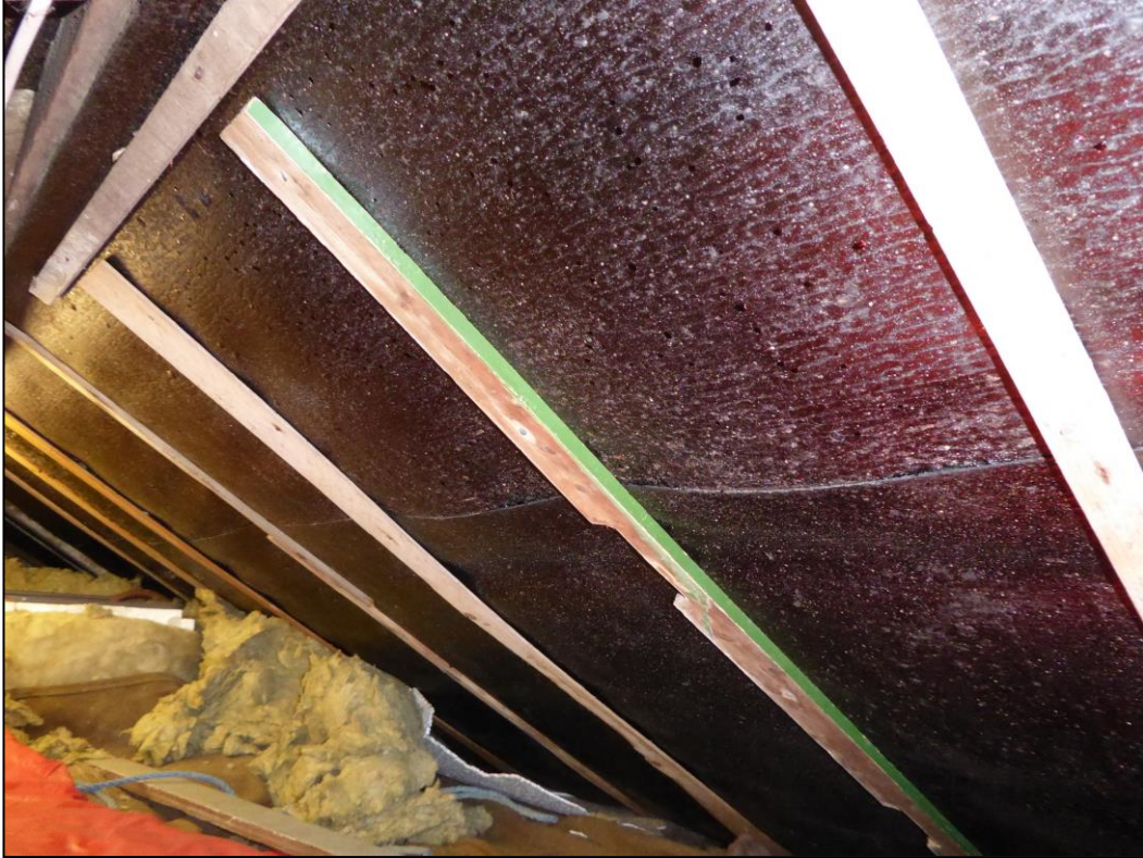
Figure 15. Example of bitumen lining, loft at 66 Chapel Hill, Tilehurst. 26.03.19
