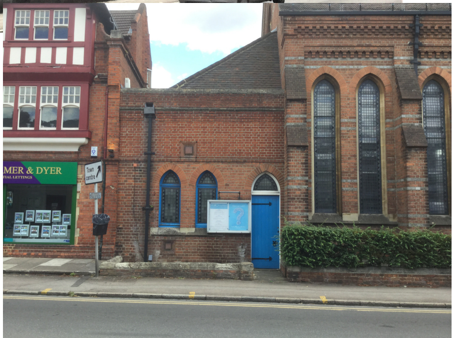
View from Prospect St- West Elevation- Rear Entrance
