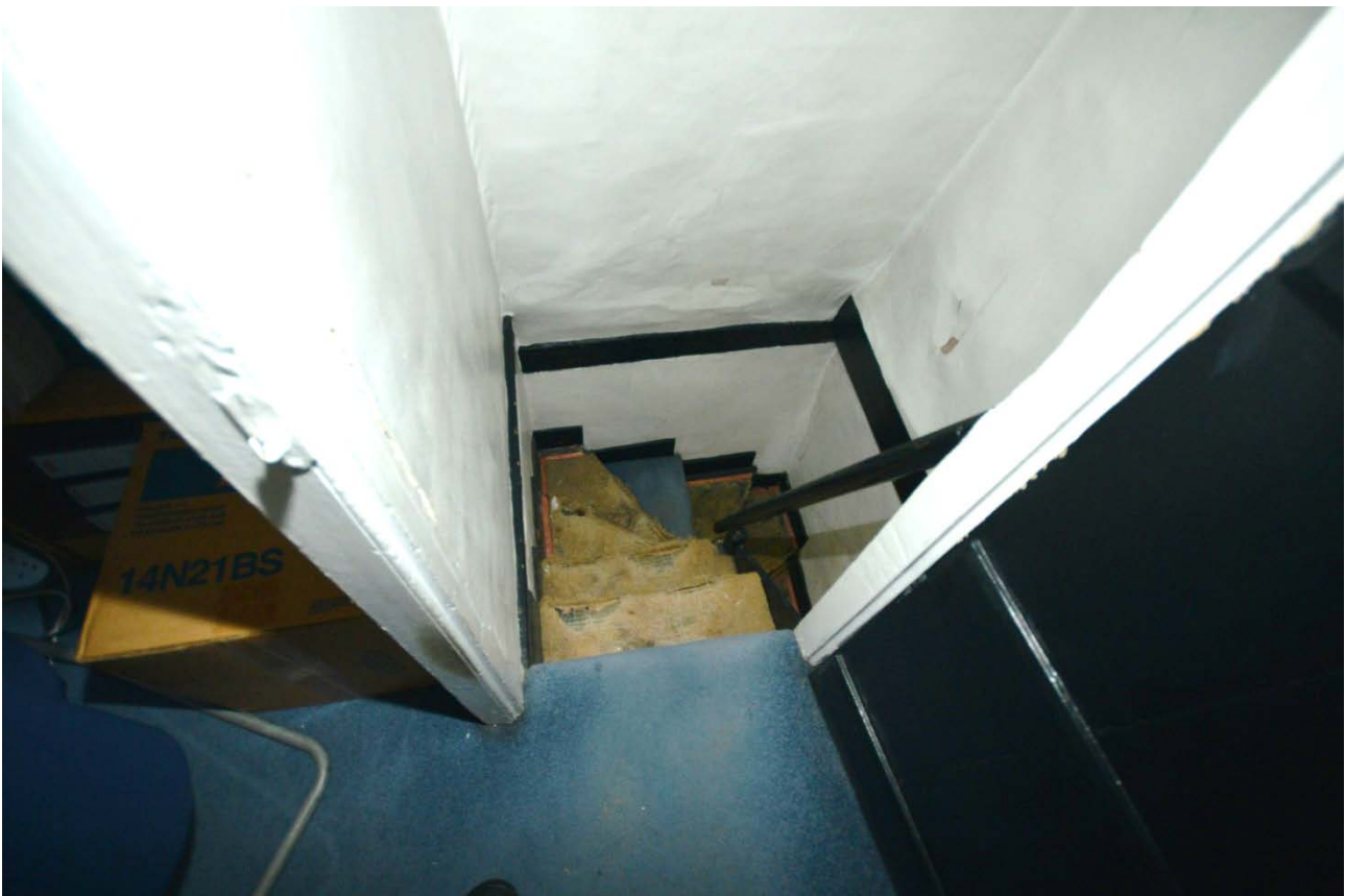
Plate 8: Staircase from first to second floor
