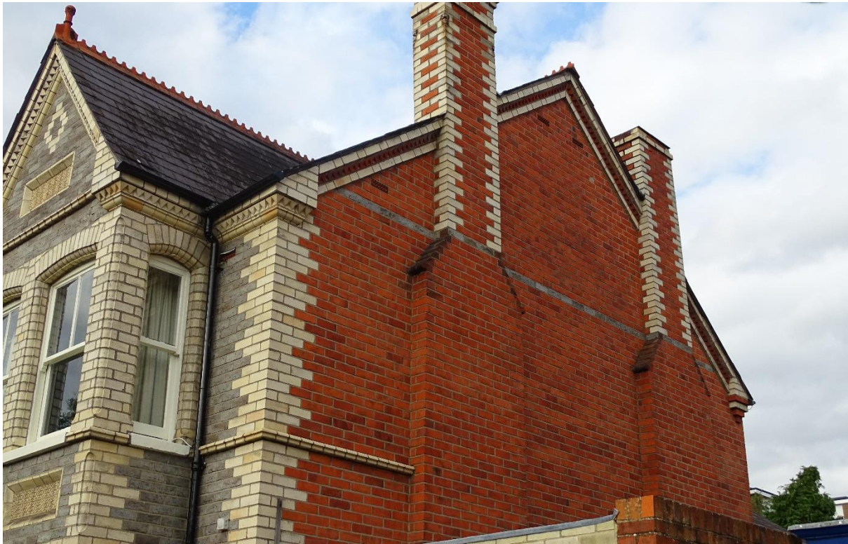
Image 3 – South facing elevation of the property
