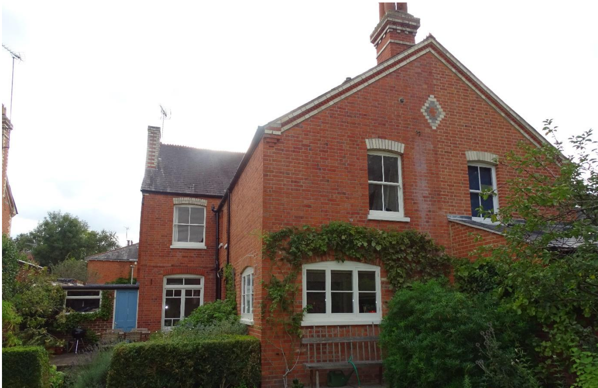
Image 4 – Rear East facing elevation of the property
