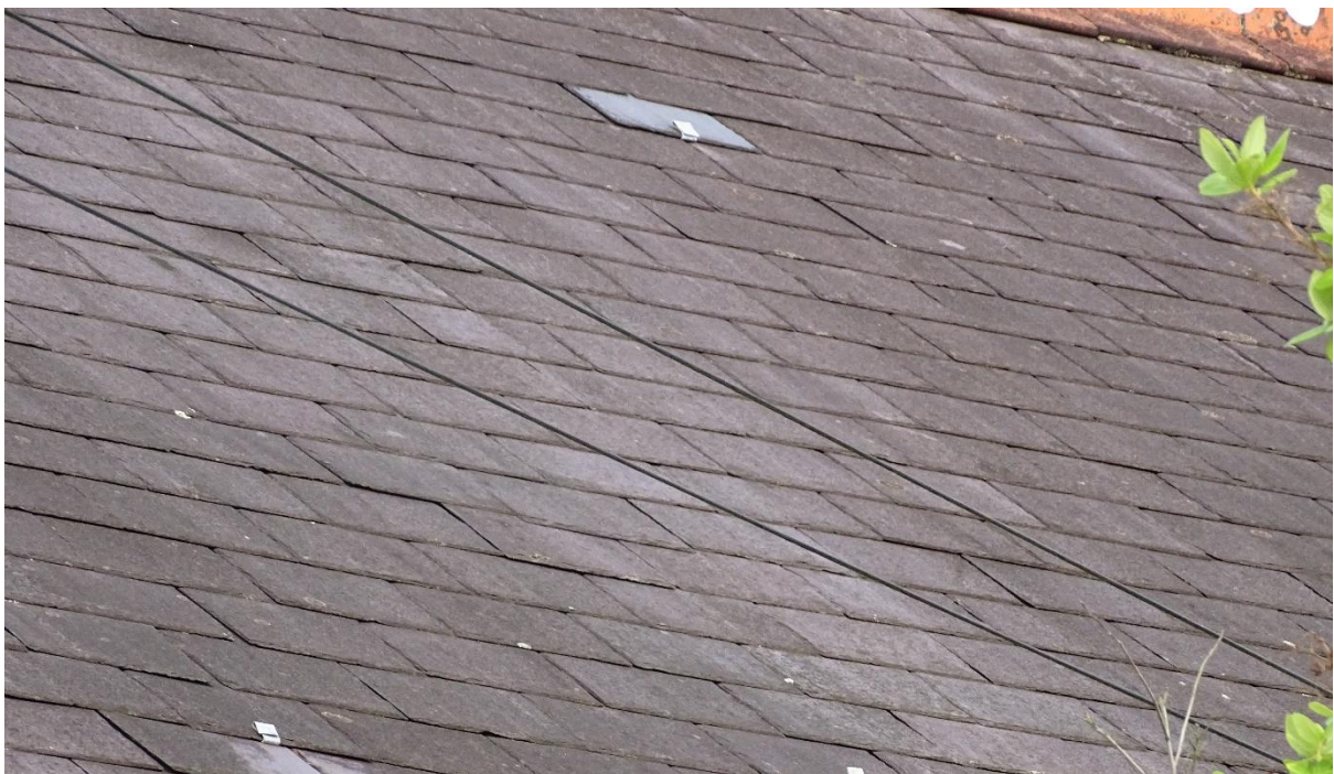
Image 2 – Close view of the roof coverings to the front West facing elevation where no features of value to bats were noted within
