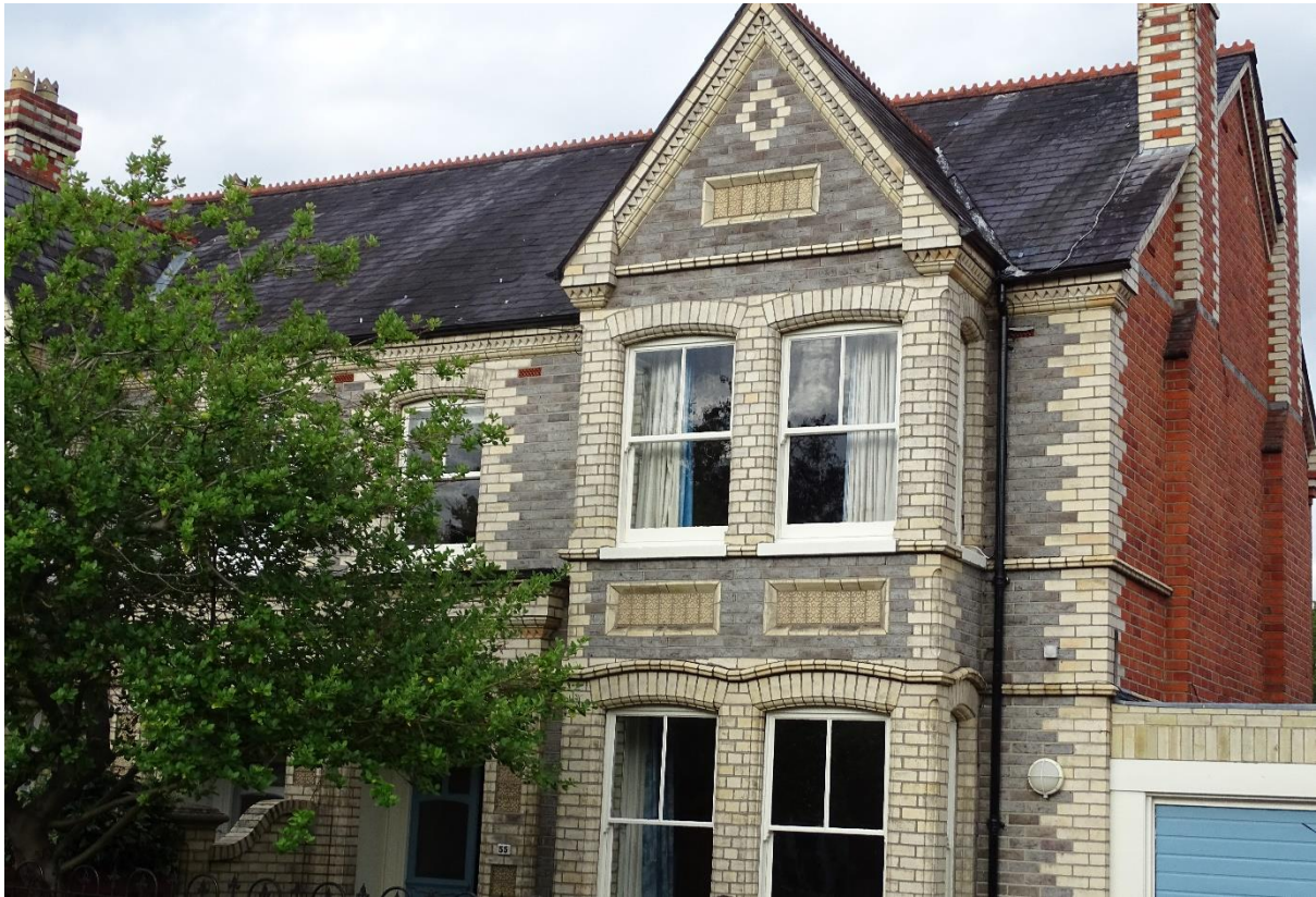
Image 1 – Front West facing elevation of the property
