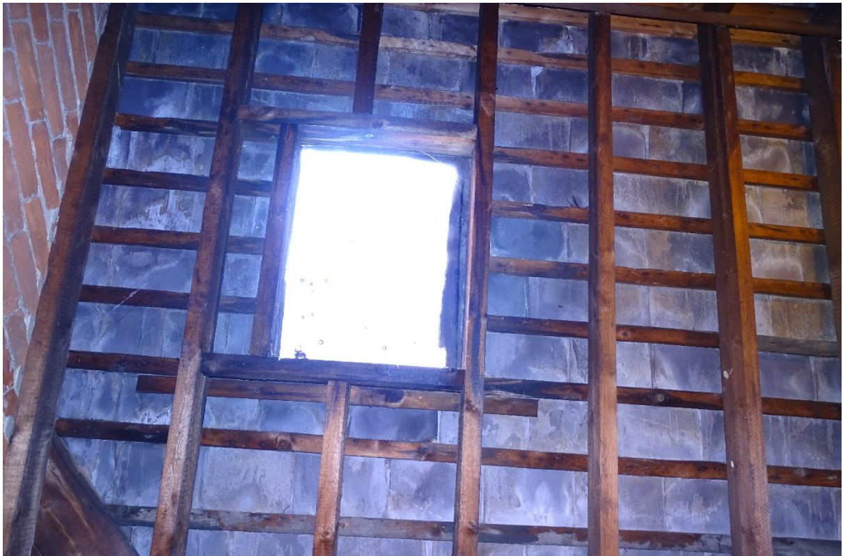
Image 7 – Roof lights within the roof coverings which offer a good level of natural lighting within the roof void spaces throughout
