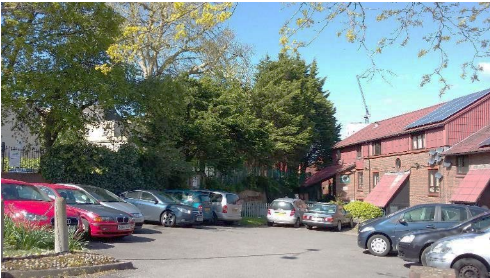
Fig 12. View of Morriss Court from Orts Road.
