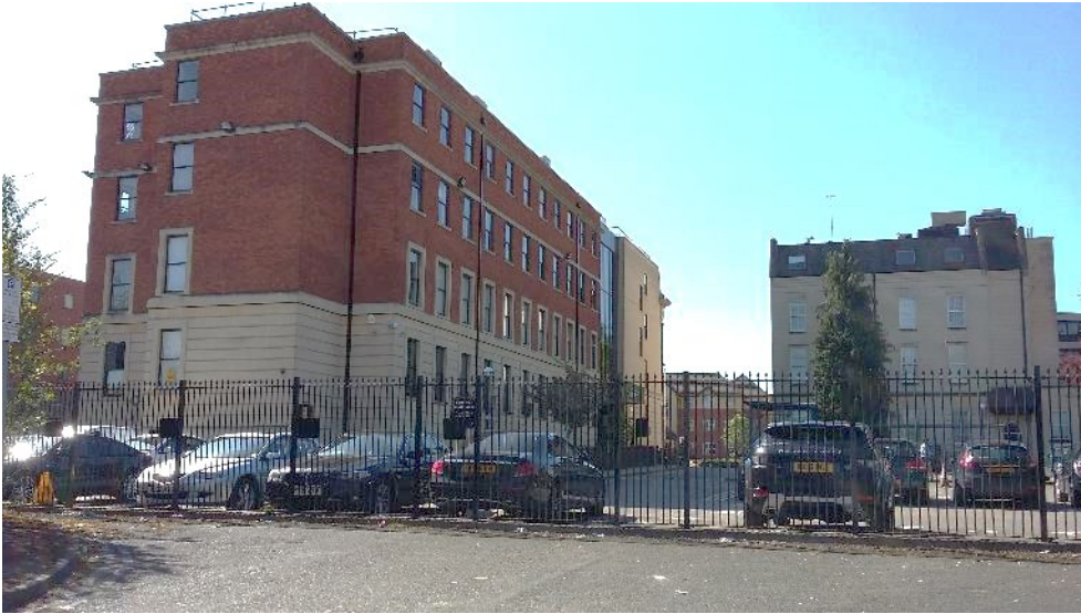
Fig 11. View of rear of 185 Kings Road.
