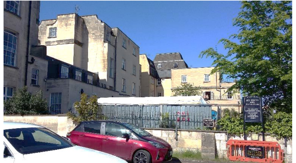
Fig 9. View of the site from the rear of 179 Kings Road.
