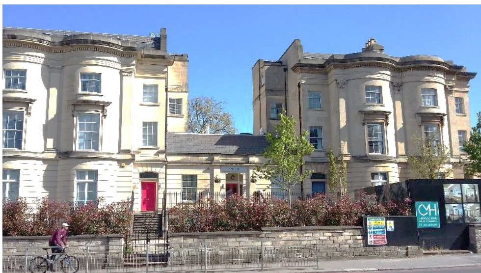
Fig 15. View of 175 and 177 Kings Road.
