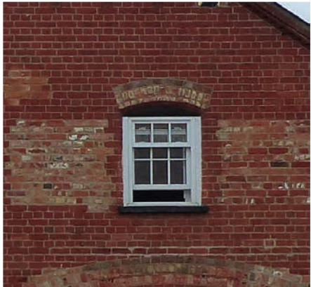
Small sash window with arch lintel
