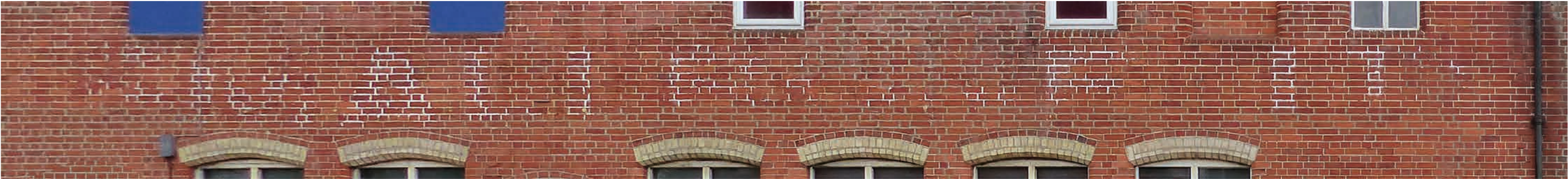
Inset brick to replicate window opening
