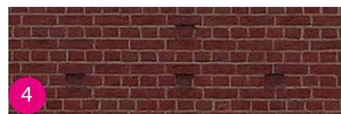
Brick detailing to the former malthouse buildings
