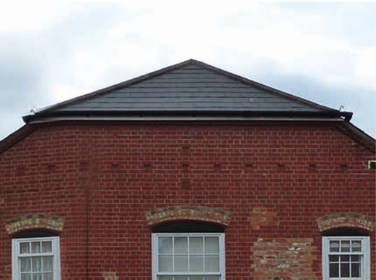
Half hipped roof forms
