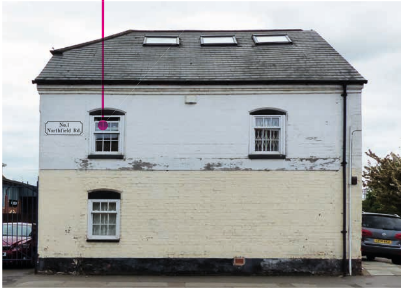
EXISTING OFFICES - FACING NORTHFIELD ROAD
