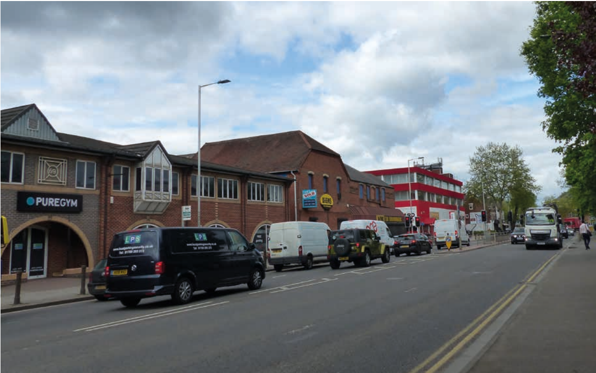
EXISTING DREWS BUILDING - VIEW FROM SOUTH OF CAVERSHAM ROAD
