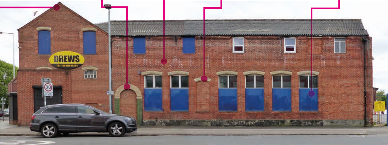
EXISTING DREWS BUILDING - NORTHFIELD ROAD FACADE
