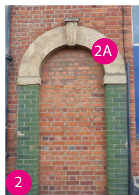
Green glazed brick arch to the Northfield Road facade
