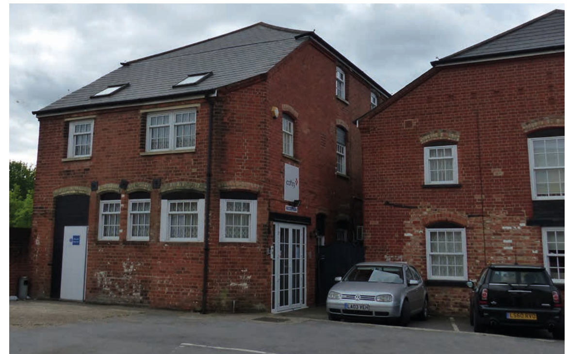
VIEW FROM CAR PARK AREA TO OFFICE BUILDINGS
