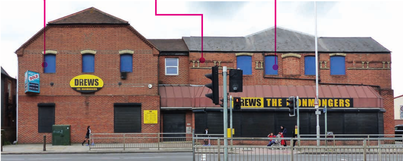
EXISTING DREWS BUILDING - CAVERSHAM ROAD FACADE
