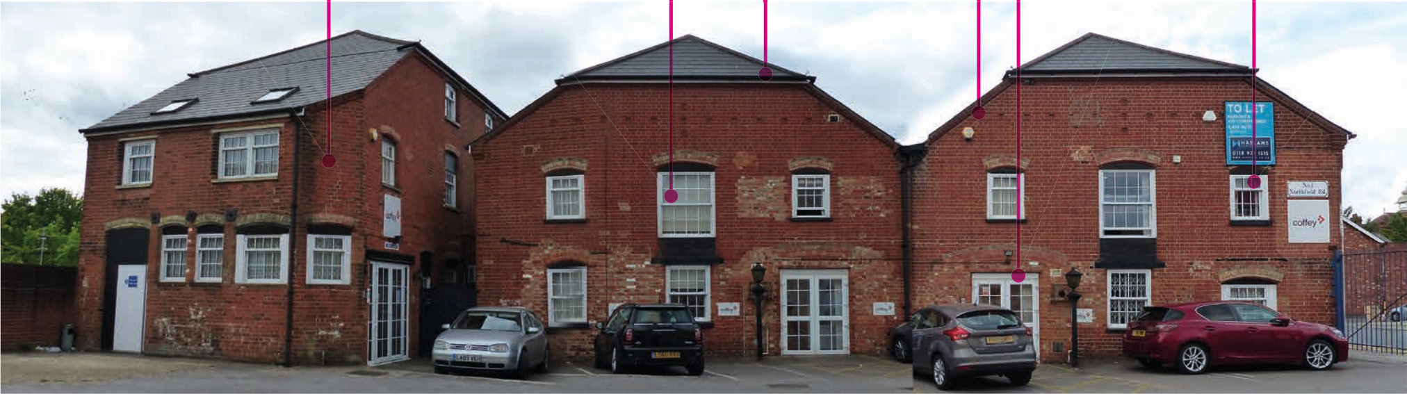
EXISTING OFFICES - FACING THE BACK OF DREWS BUILDING
