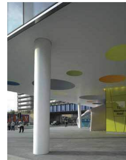
Southwark: dramatic undercroft signals a special place in the local urban hierarchy
