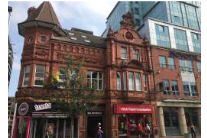
Late Victorian/Edwardian building on Friar St to the east of the site
