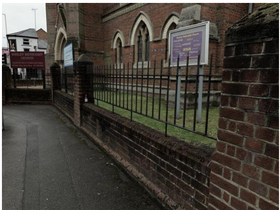
Existing railings to Wesley Methodist Church
