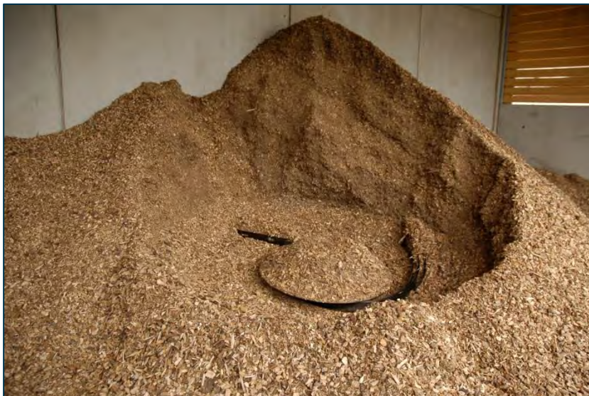
Figure 7.7: Biomass fuel (wood chips) in a storage hopper
