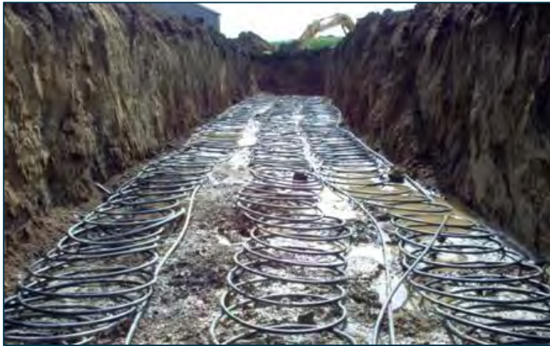
Figure 7.4: Ground source heating horizontal collector loops being installed
