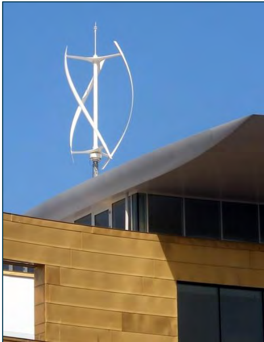
Figure 7.5: A roof-mounted wind turbine
