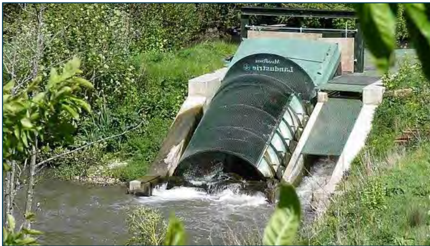
Figure 7.6: An Archimedean screw hydropower scheme
