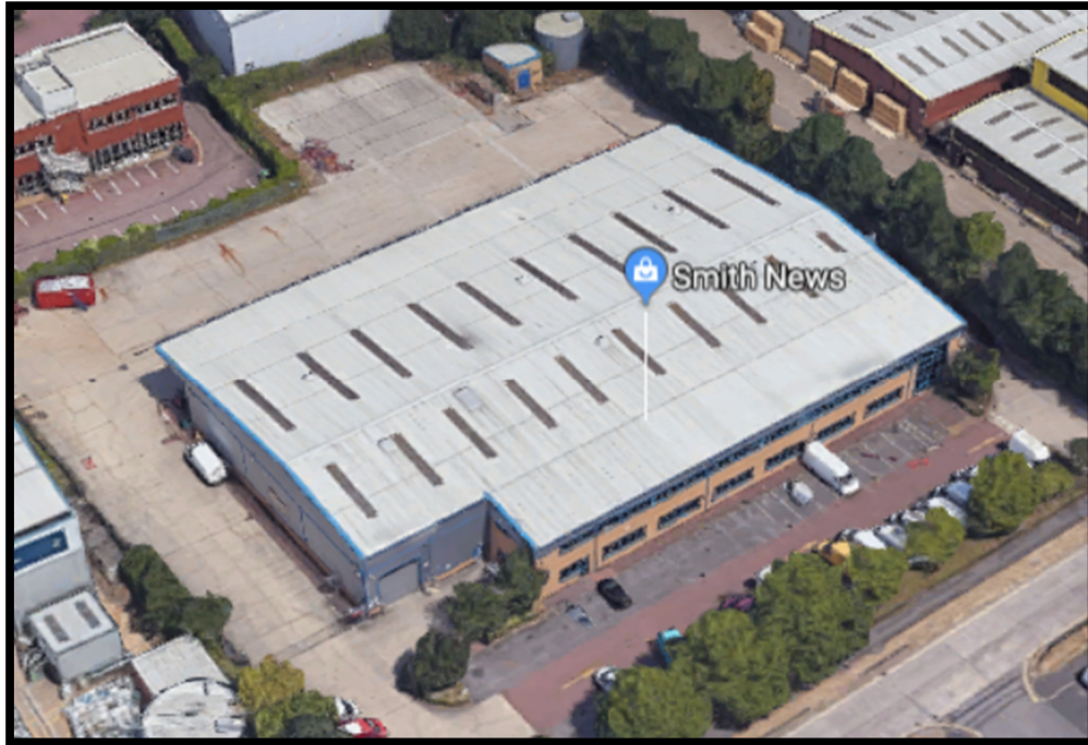
Aerial view of 4 Acre Road
