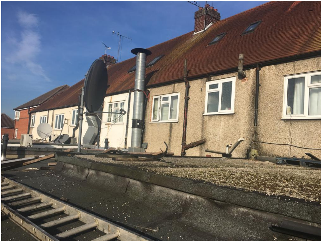
The plant machinery of the extraction kitchens of the kebab shop and chinese takeaway.
