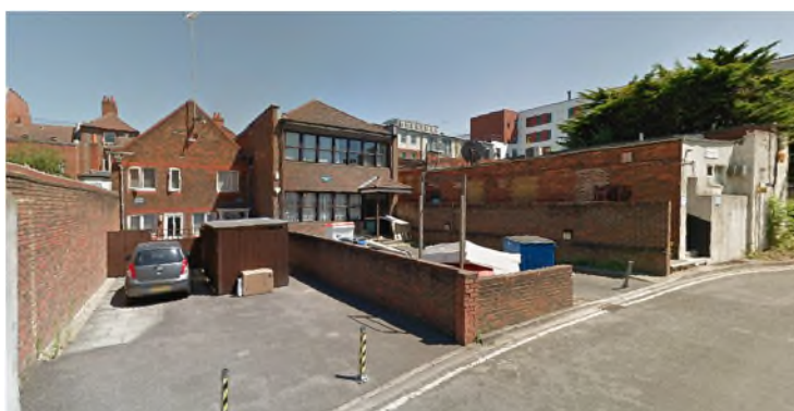
Figure 5: Poor quality extensions to London Street properties with Prince Regent House at the centre of the image
