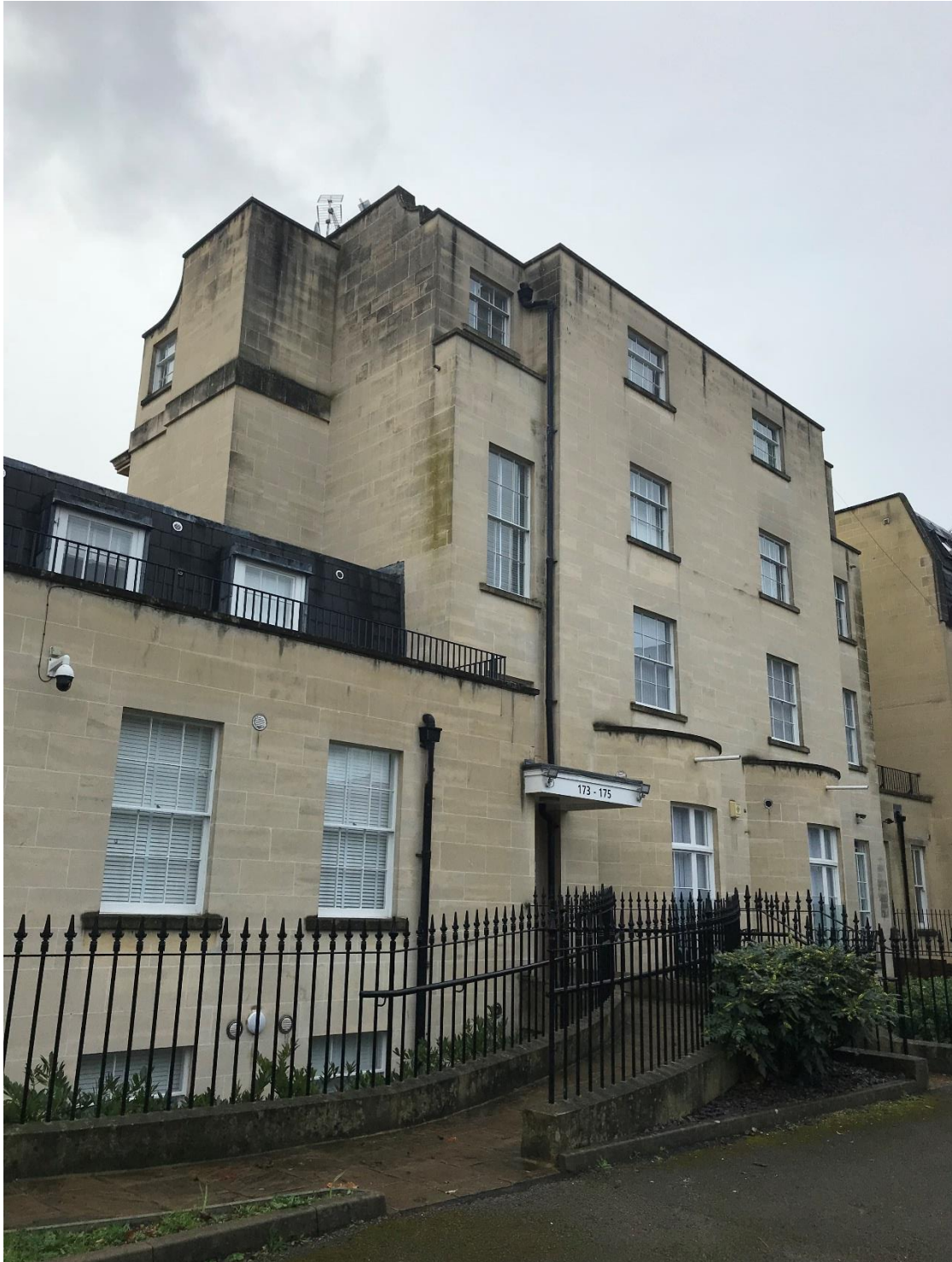
Figure 9 – Rear of 173/175 Kings Road. The back of this pair has been entirely rebuilt.
