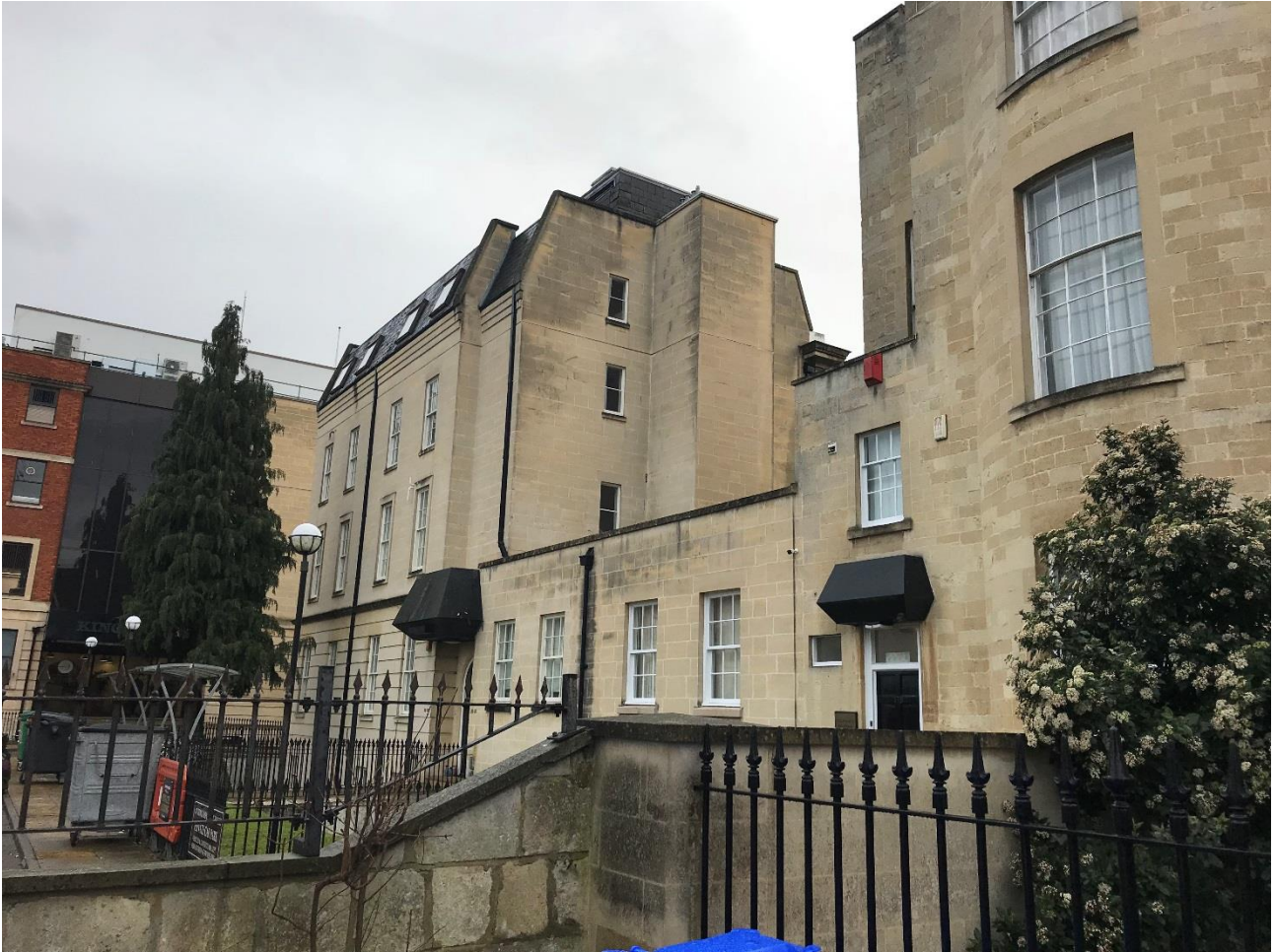
Figure 10 – The rear of 181/183 Kings Road. The rear of this pair has also been entirely rebuilt.
