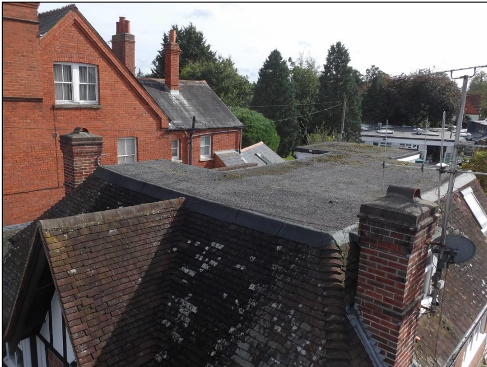
Figure 3. Example of roof structure. 11 Holmes Road, Reading. 09.10.19
