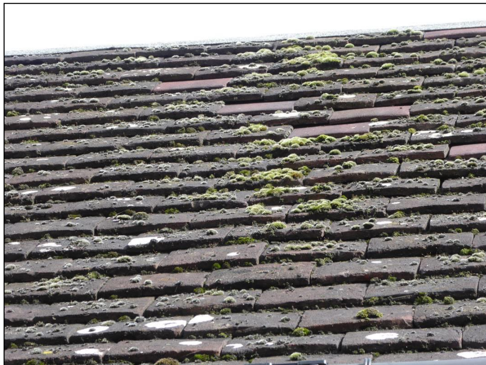
Figure 4. The roof tiles. 11 Holmes Road, Reading. 09.10.19
