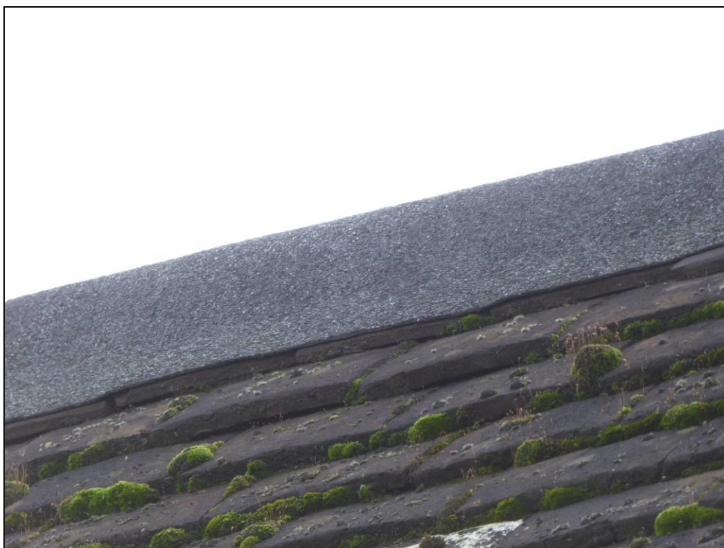
Figure 6. Example of roof joint between pitched and flat roofs. 11 Holmes Road, Reading. 09.10.19
