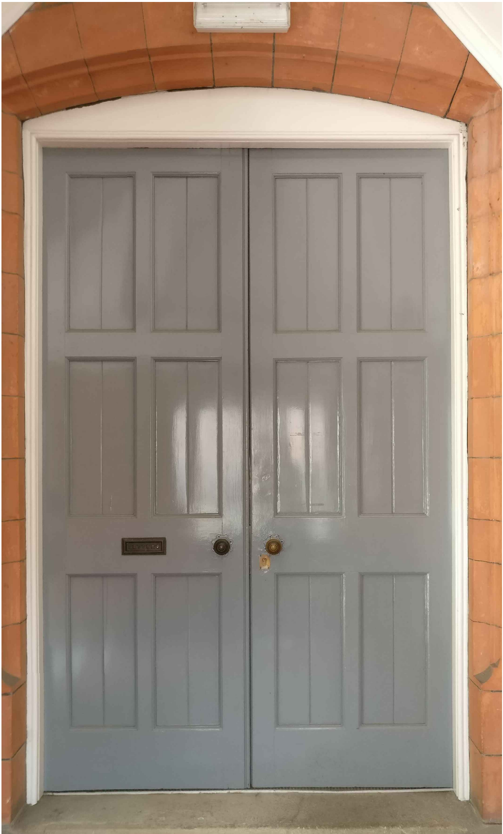
External Existing Photograph
