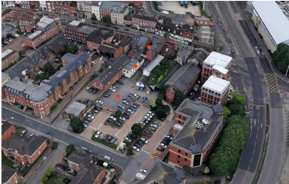
Aerial view of the site – rear parking area, 43a and 43 London Street
