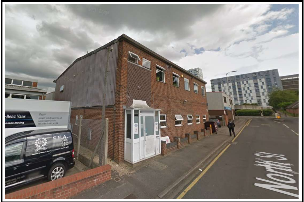
Existing Building from North Street
