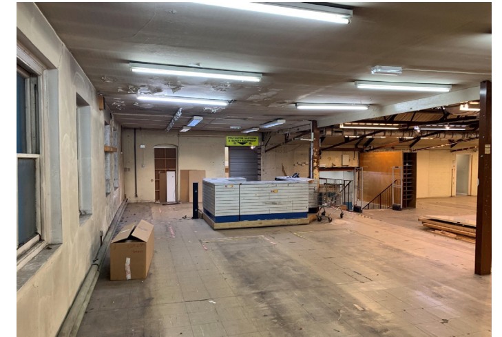
Figure 4.3 Interior of main building, first floor
