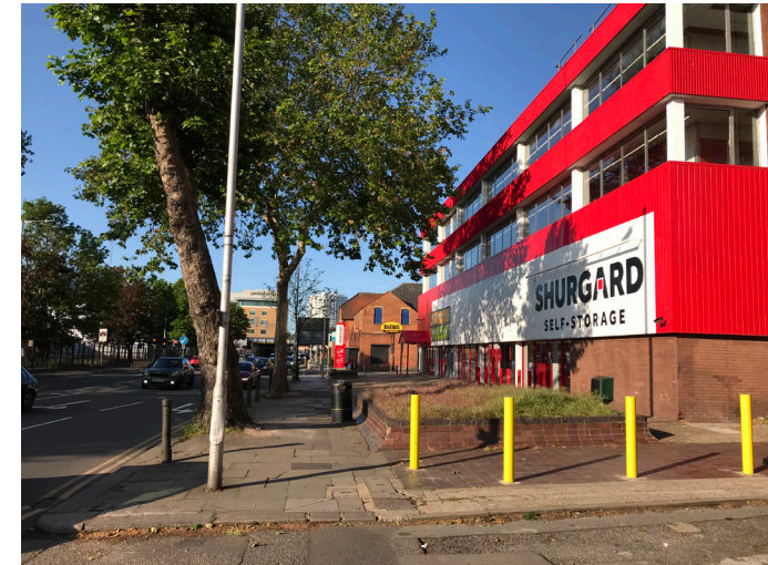
Figure 4.7 Warehouse building to North of the Site, June 2019
