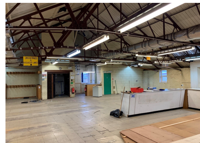
Figure 4.2 Interior of main building, first floor
