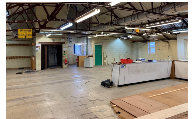
Figure 4.6 Interior of main building, first floor
