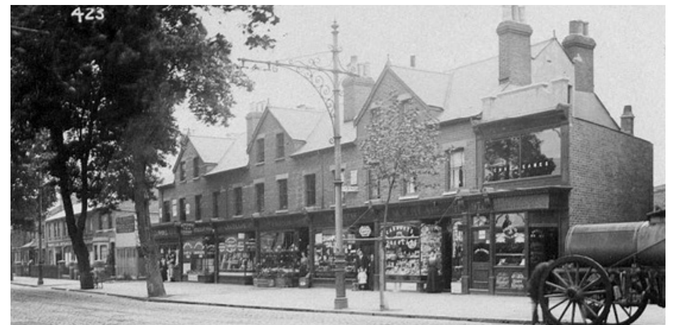
Figure 3.8 Historic image of Caversham Road
