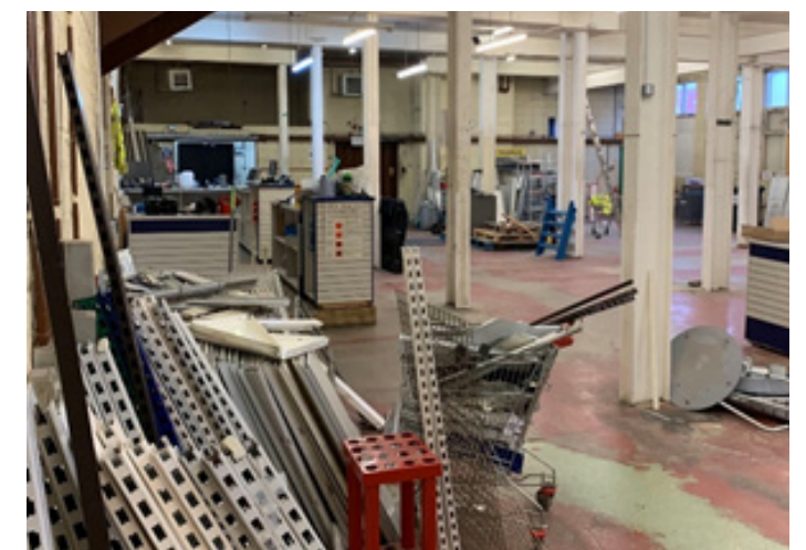
Figure 4.4 Interior of main building, first floor
