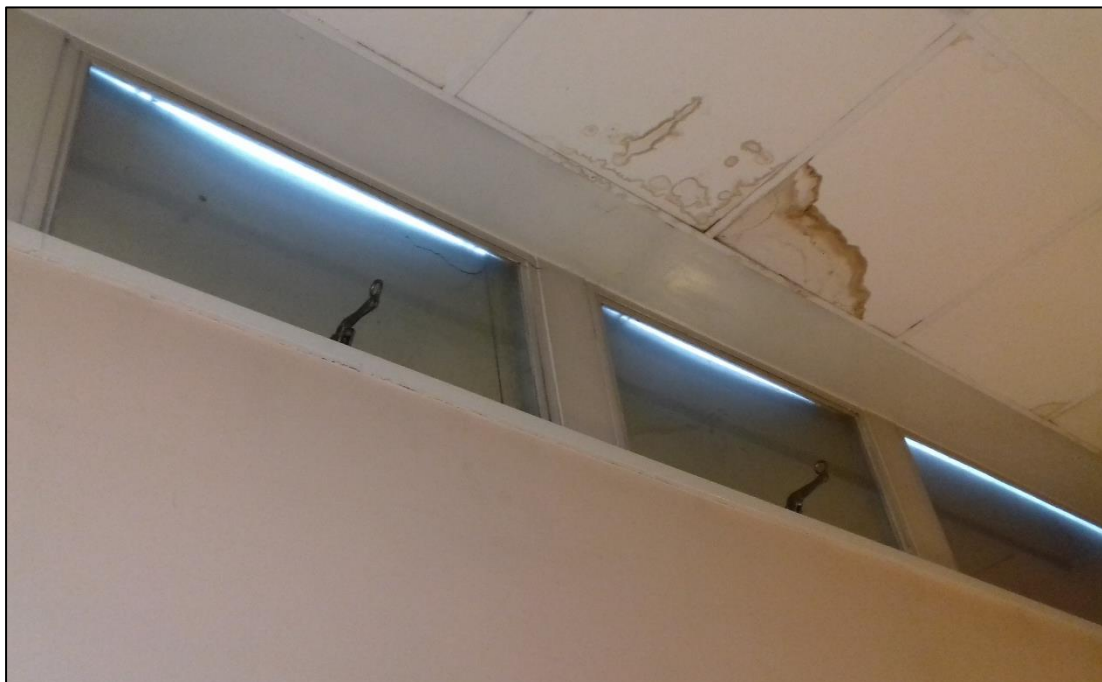
Figure 8: Interior of the Hamilton Centre
