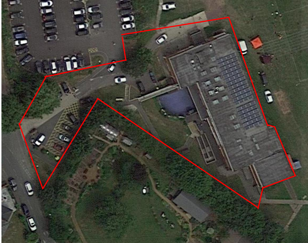
Figure 3: Surveyed area of site (red outline)
