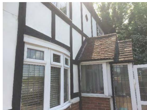
Photo 6: West aspect showing roof of front porch.
