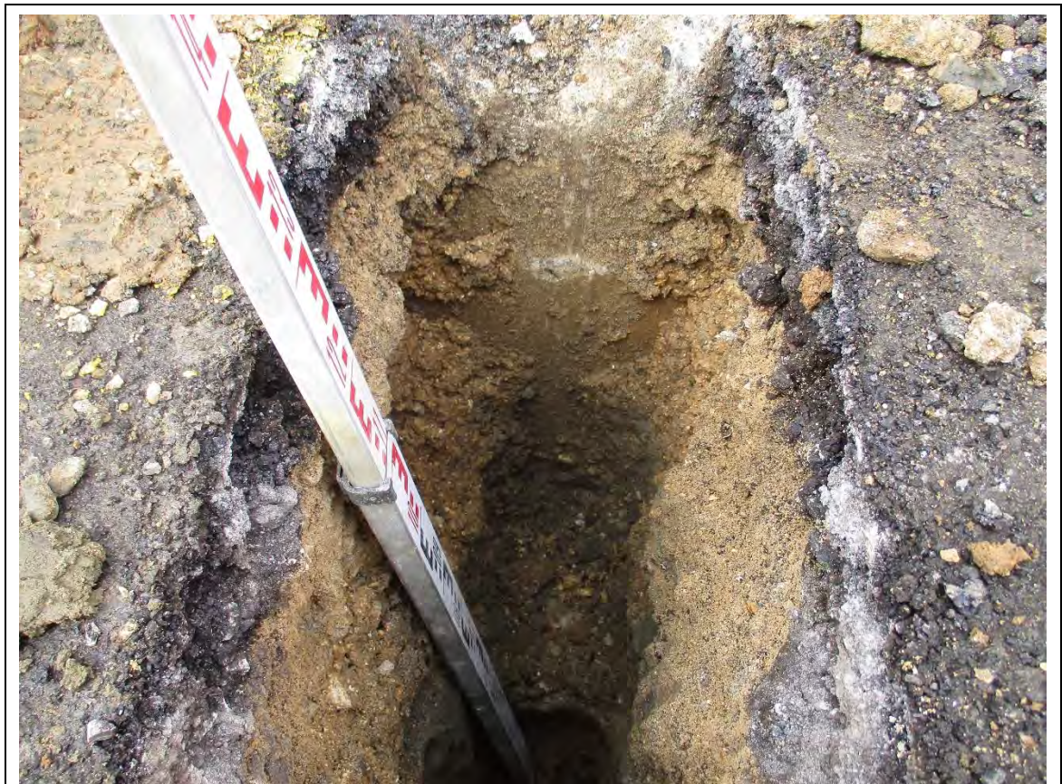
Inspection pit: IP02 profile
