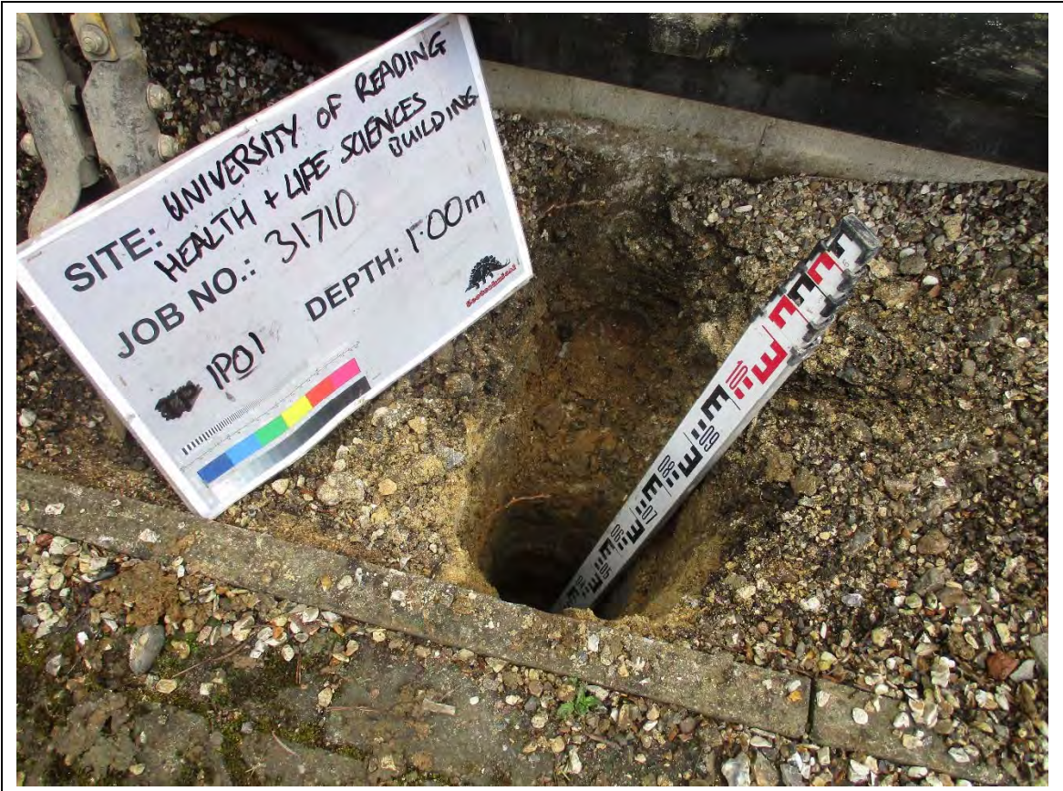
Inspection pit: IP01
