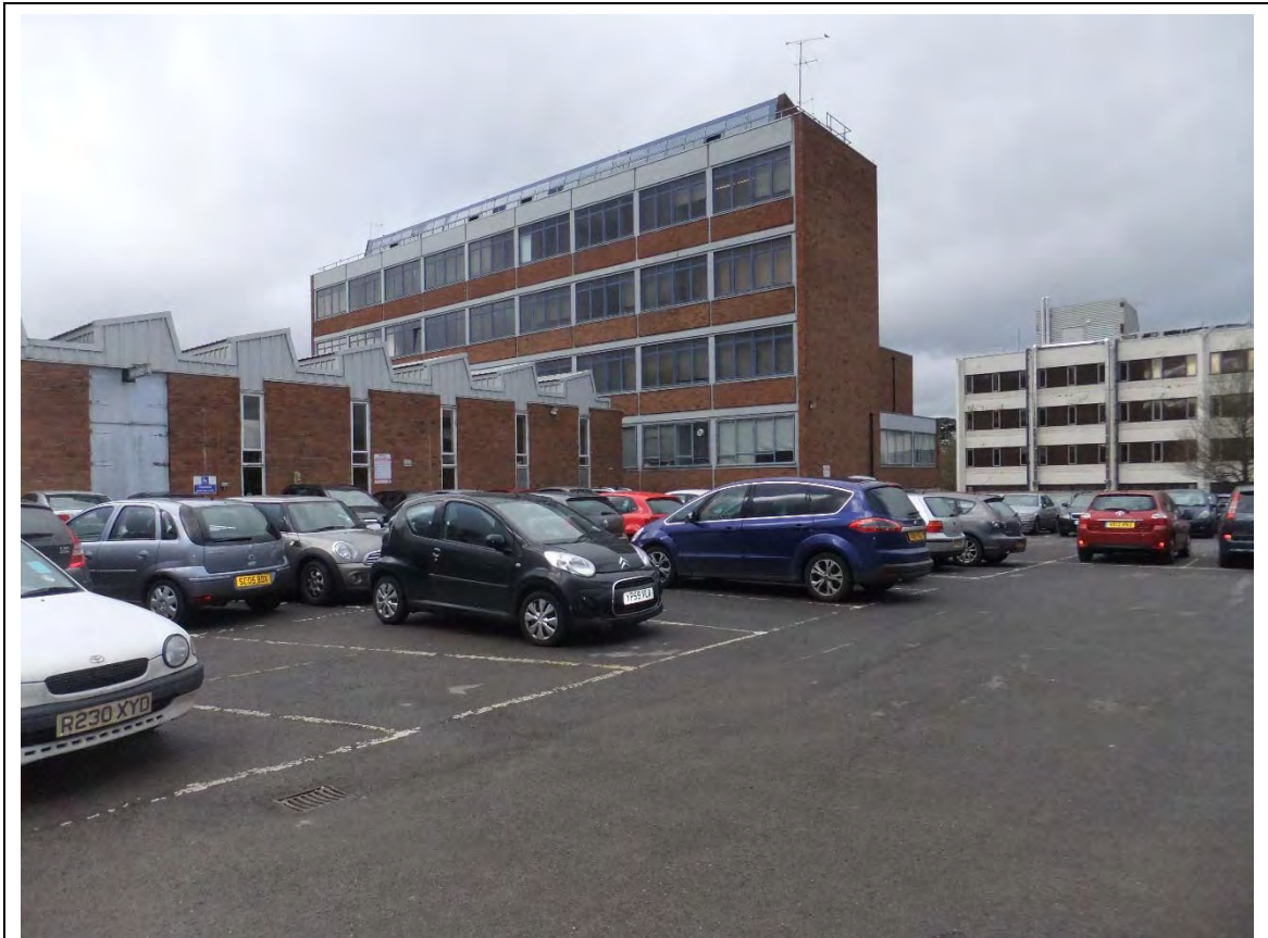
View across Car Park 12, looking northwest towards the Engineering Building
