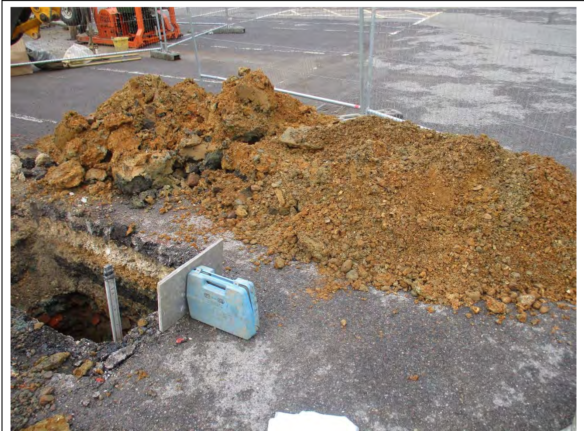
Trial pit: TP02 spoil
