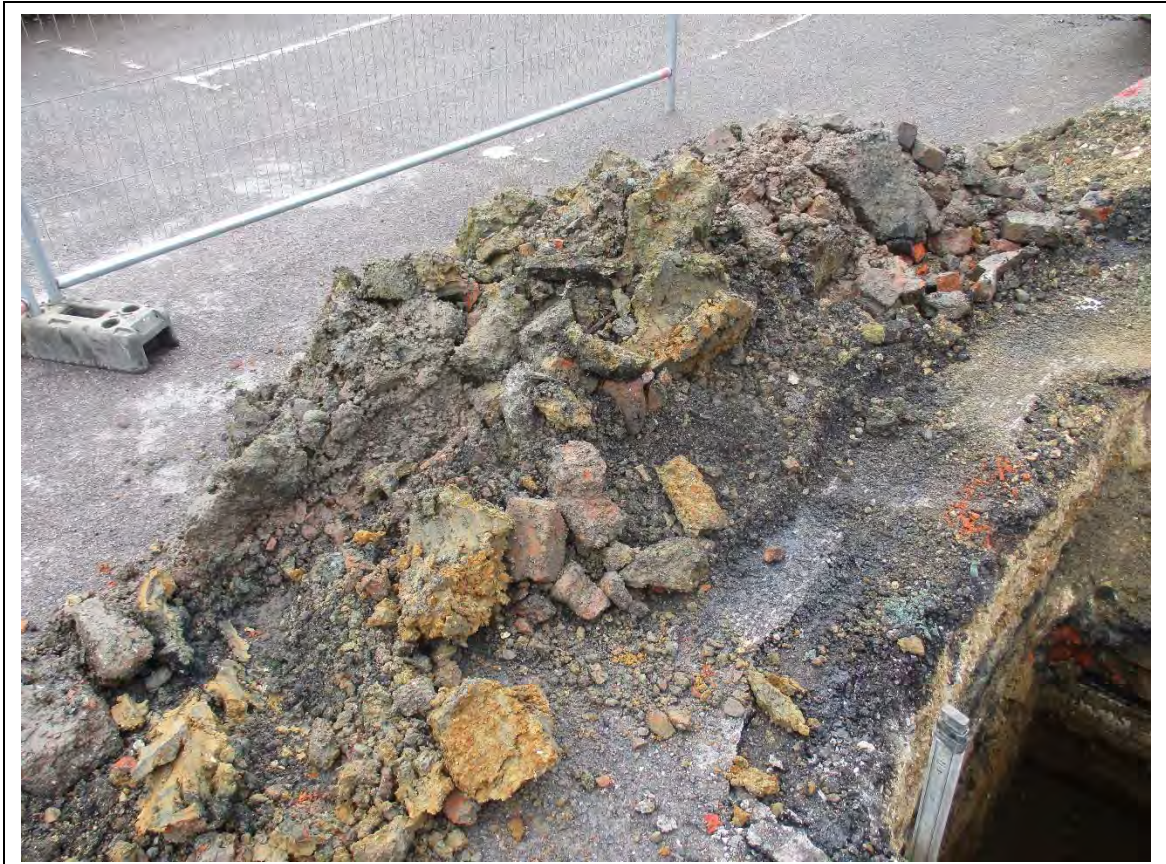
Trial pit: TP02 spoil
