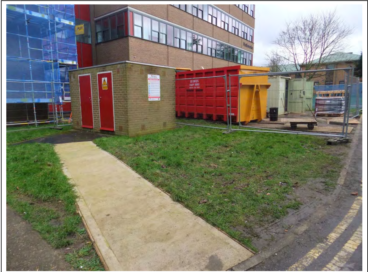
Site of the proposed substation, adjacent to the JJ Thomson Building
