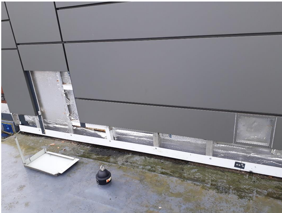
Panels removed A147, H103, H105, H107 and part H107 above.
