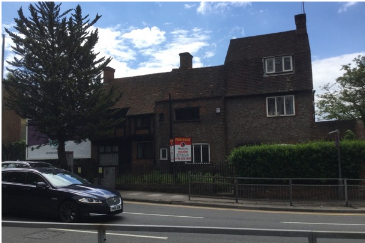
Photograph 1. The east facing elevation of building at 26-28 Southampton Street.
