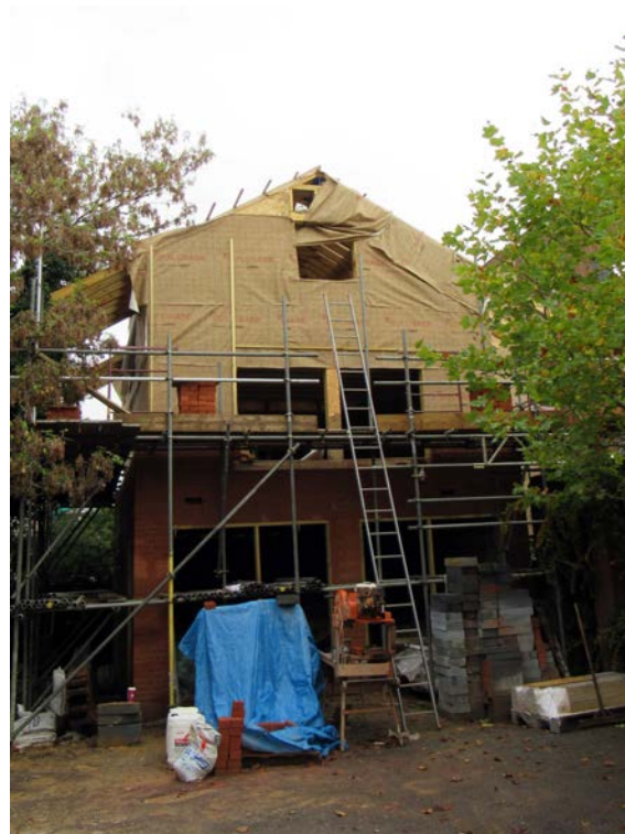
Fig.2: Current photograph of Annex building with construction work on hold
