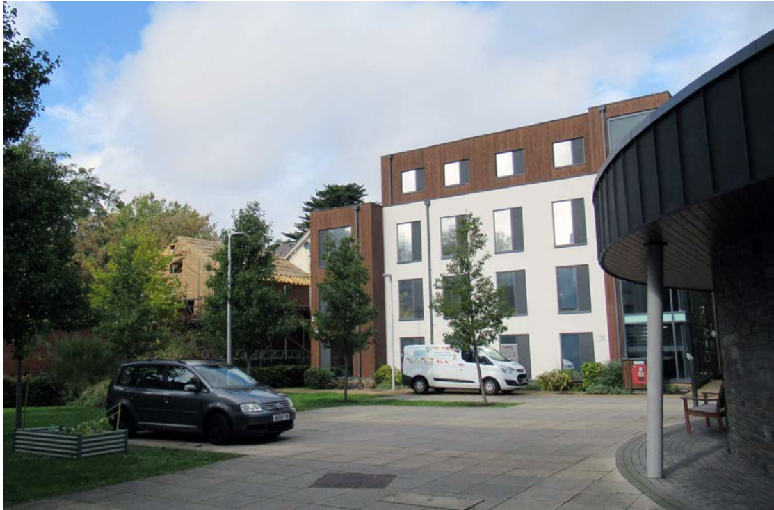
Fig.5: Photograph of Unite (Kendrick Hall) student housing blocks located to the east
