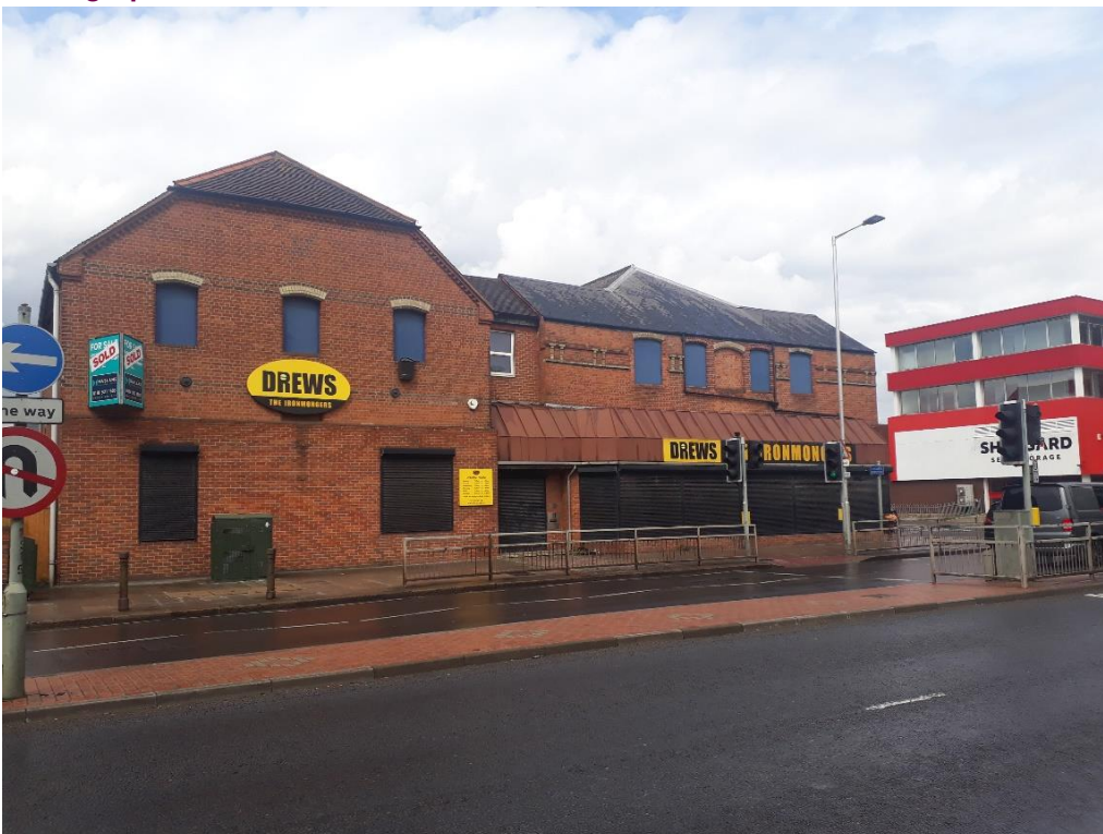
Photograph 2: Front of 71-73 Caversham Road
