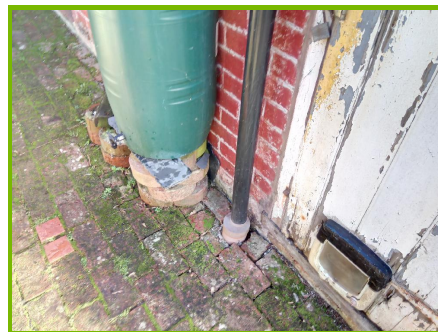
Fig 1.3: Rain water pipe 1
