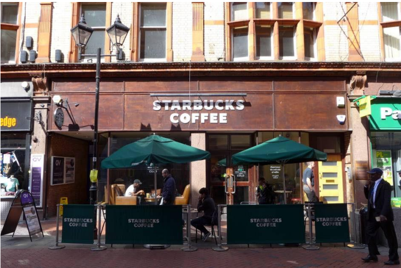
View of the Front of the Building
