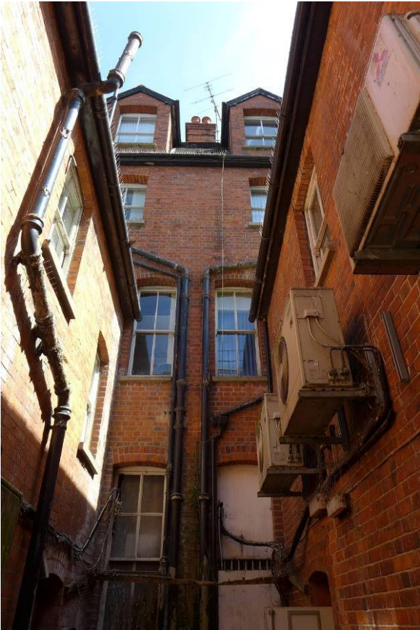
View of the Rear of the Building
