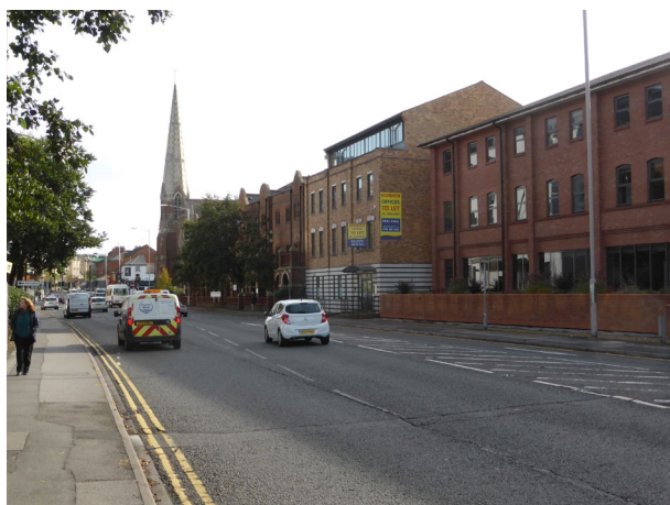
View of Queens Road, showing the adjacent taller Havell House, with set-back upper floor, and Wesley Methodist Church in the background
