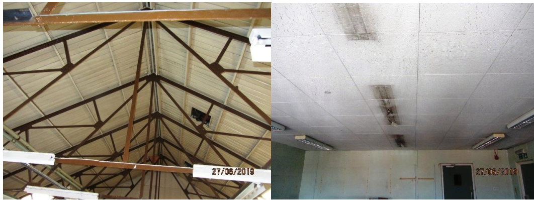
Photographs 7 - 8: Internal roof spaces (two rear extensions)
