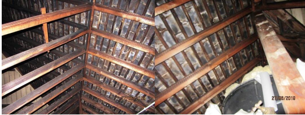
Photographs 5 - 6: Internal roof spaces (fronting Cavendish Road)
