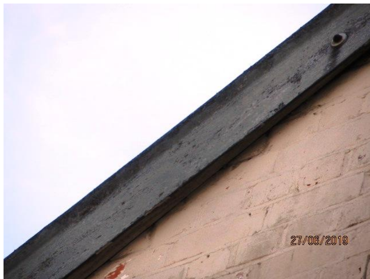
Photograph 9: Close-fitting soffits / barge boards
