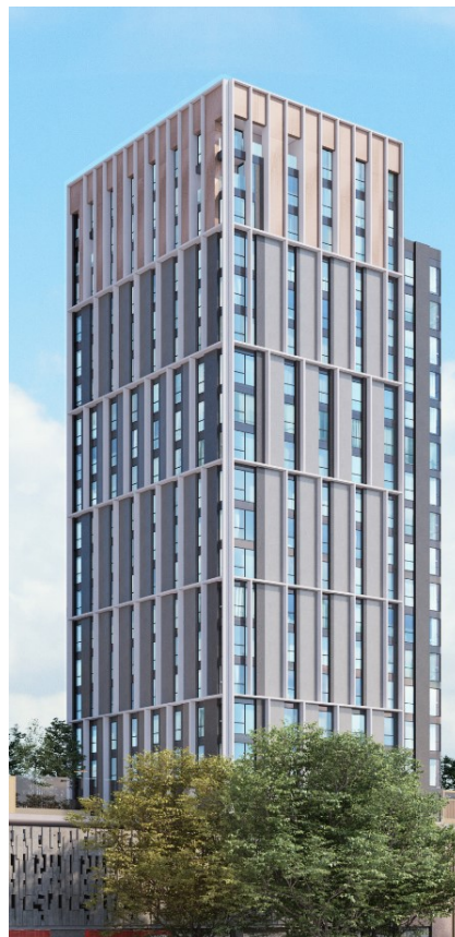
Figure 4.13 Appearance of Building B
