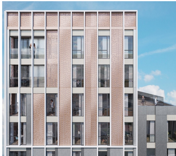
Figure 4.12 Appearance of Building A
