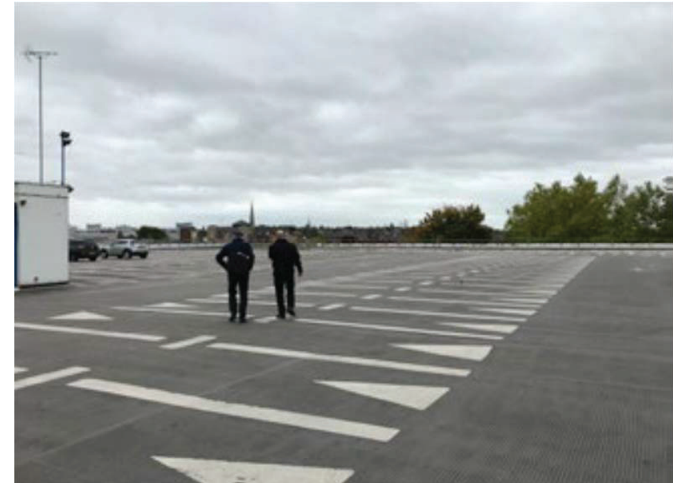
Figure 3 Second Storey Roof Car Park, above the Broad Street Mall
